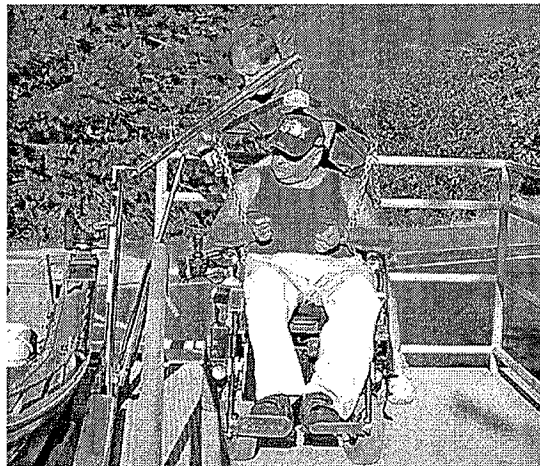
Accessible loading platform and slip for a patient lift at Centimudi public boat ramp at Shasta Lake.
