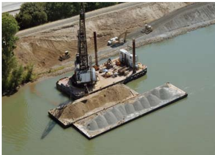
Levee repair site on Sacramento River
