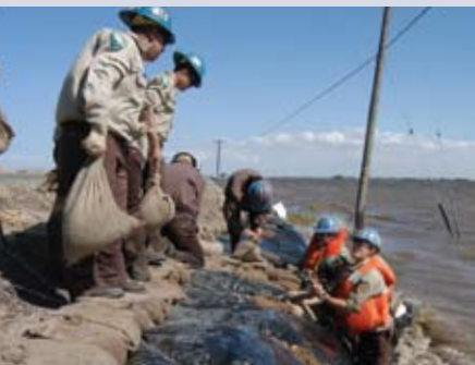
California Conservation Corps workers strengthen a levee during a high water event
