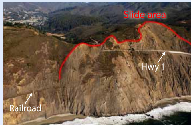
The Devil's Slide area near Pacifica, CA (south of San Francisco) shows remnants of a destroyed rail line, as well as modern California Highway 1. The area has experienced repeated sliding over the years. Photo copyright (C) 2002-2012 Kenneth & Gabrielle Adelman, California Coastal Records Project, www.Californiacoastline.org.
