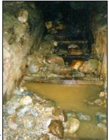
Tunnel sluice with mercury-contaminated sediments.
