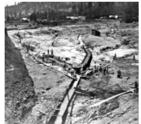
Figure 3. Gravel deposits were washed into sluices (from center to lower part of figure) where gold was recovered.
