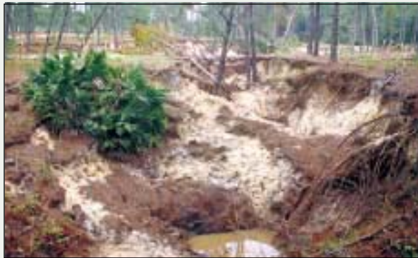
Figure 19. Human-induced sinkholes formed during the development of an irrigation well affected a 20-acre area and ranged in size from less than 1 foot to more than 150 feet in diameter. (Photograph courtesy Ann Tihansky, USGS.)
