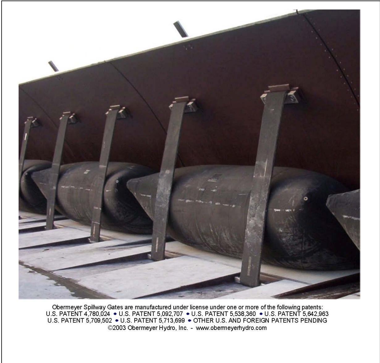
Figure 1 Typical Obermeyer Gate
