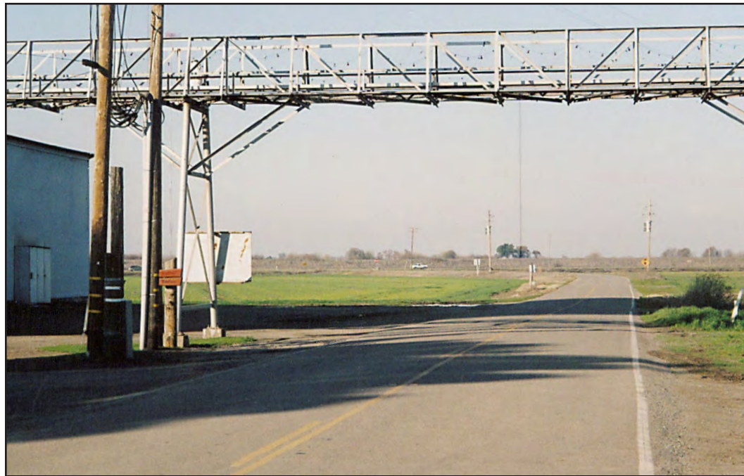
Figure 5.5-16. View of Staten Island Road, looking northeast toward intersection with Walnut Grove-Thornton Road (at stop sign visible at center of photo, being approached by white truck). The grain dryer facility is partially visible at left. KCRA-3 transmission tower is faintly visible in background at right center of photo. This area is subject to modification under Alternatives 2-A through 2-C.
