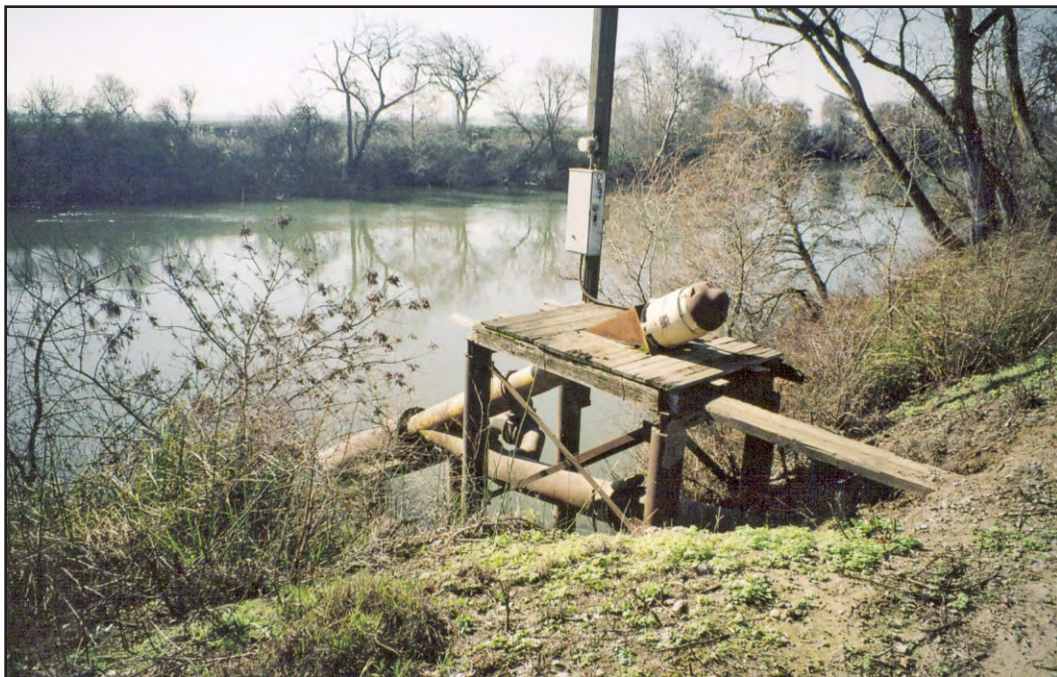
Figure 5.5-12. View of McCormack-Williamson Tract, looking south from east levee (waterside). Note irrigation siphon in foreground, pumping irrigation water from the Mokelumne River. Also note mature vegetation on the waterside of the levee. The siphon and vegetation are subject to modification under Alternatives 1-A through 1-C.
