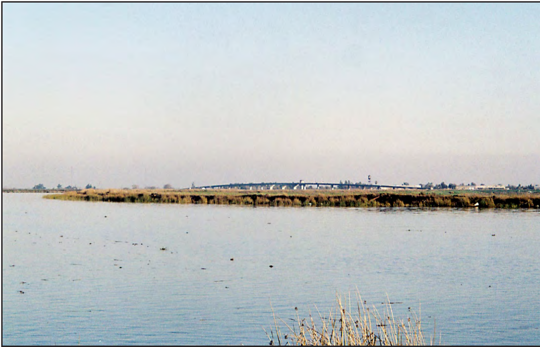
Figure 5.5-17. View of SR 12 bridge at community of Terminous, looking southeast from south levee of Staten Island. Note South Fork Mokelumne River in foreground. This levee and the corresponding levee on the opposite bank would be subject to modification under Alternative 2-D.
