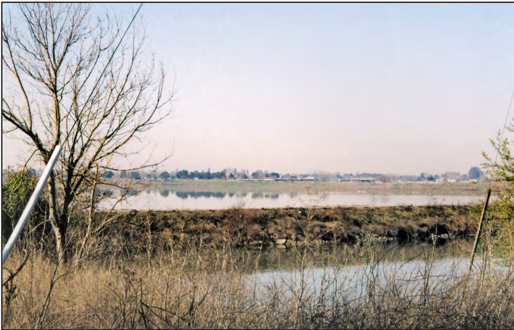
Figure 5.5-14. View of Dead Horse Island (flooded area between the levees running through the middle of the photo), looking west from the southwest levee of McCormack-Williamson Tract. Note east levee in foreground, which would be armored under Alternatives 1-A through 1-C. Controlled winter flooding (such as seen here) serves to decompose crop stubble, balance hydrostatic forces on the levee, and provide habitat.
