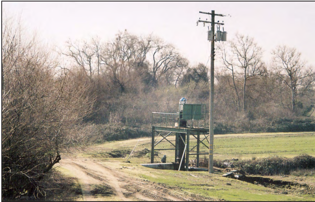
Figure 5.5-11. View of McCormack-Williamson Tract, looking south from east levee (land side). Note drainage pump station at southern end of the tract in foreground, pumping return water to the Mokelumne River. Also note mature vegetation on the land side of the levee. The pump station and vegetation are subject to modification under Alternatives 1-A through 1-C.
