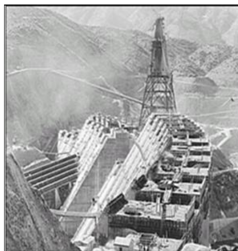
Shasta Dam Under Construction
