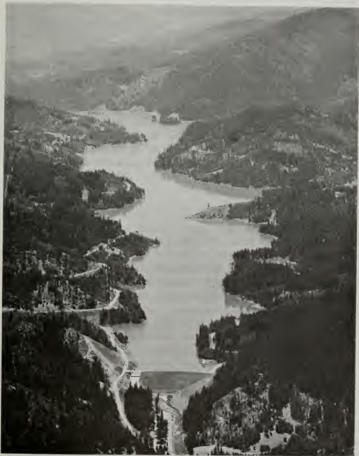
Ruth Dam and Reservoir (Courtesy Swanlund Photo Lab, Eureka, California)
