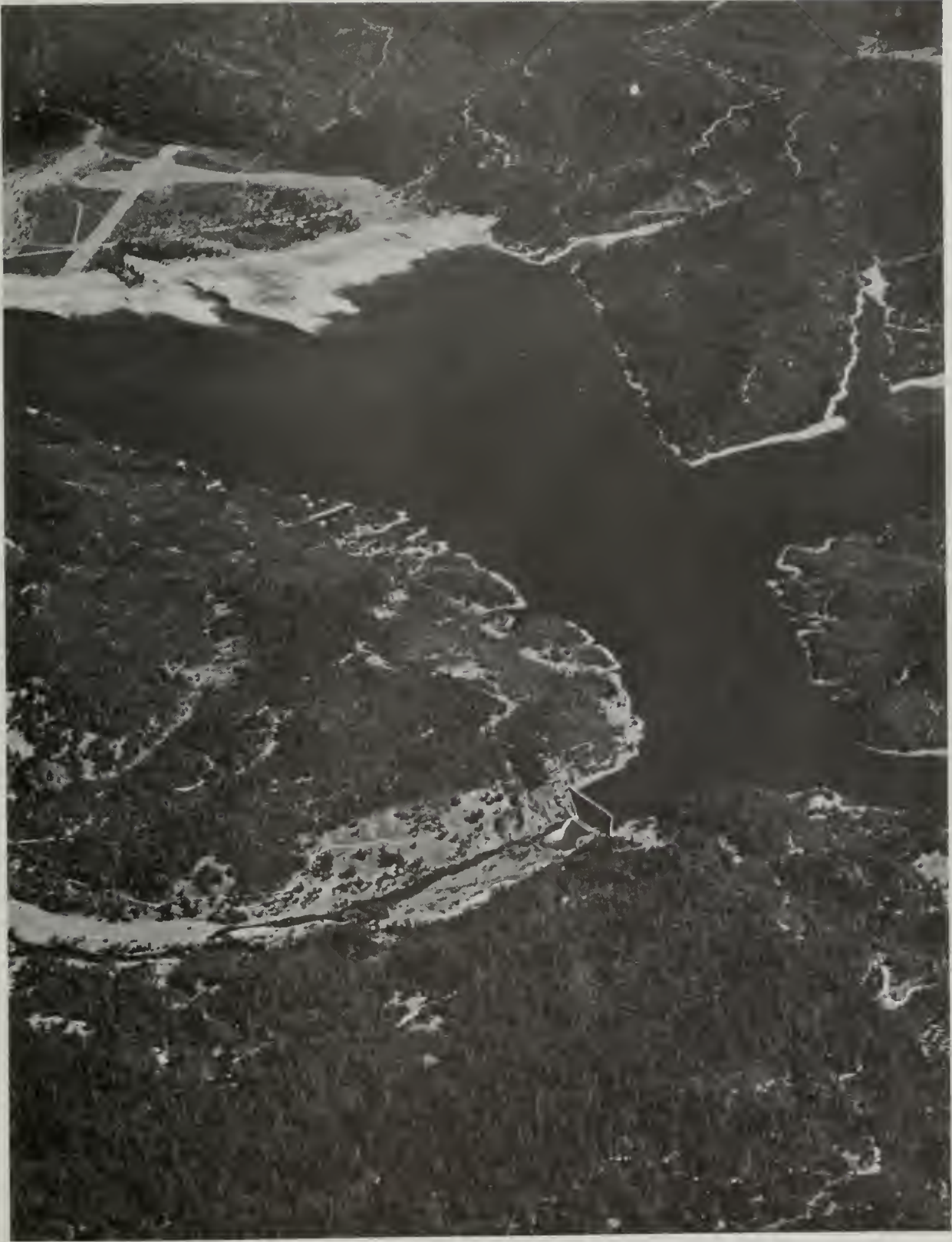
Scott Dam and Lake Pillsbury
