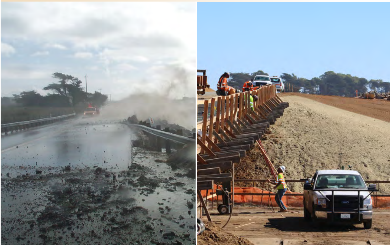
Images provided by the California Department of Transportation.
