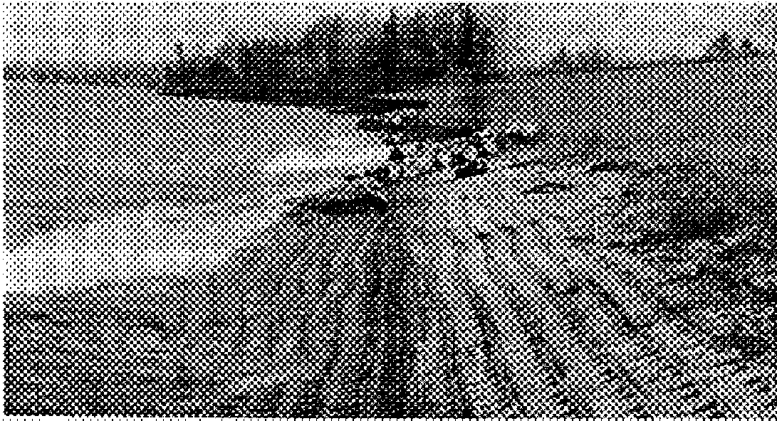
Figure B-24. Concrete control block revetment, Port Wing, WI
