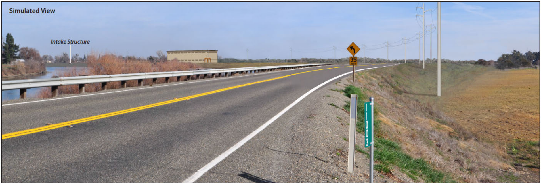
Figure 17-78 Existing and Simulated Views of Intake 4 East from SR 160 (Alternatives 1A, 1B, 2A, 2B, 6A, and 6B)
