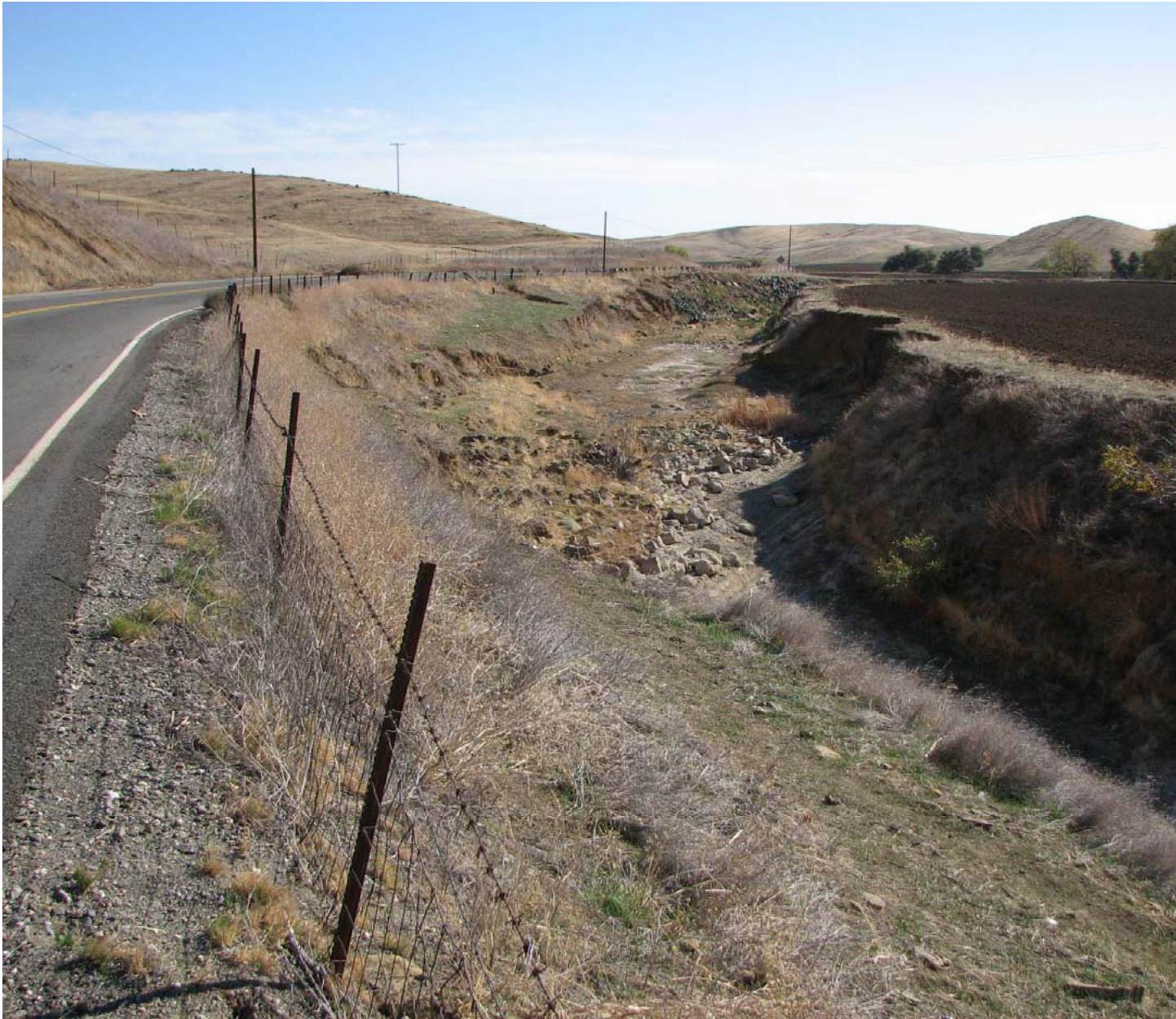
Figure 6-Geomorphology. Photo of Stone Corral Creek looking approximately upstream and downstream from edge of Maxwell Sites Road about 3 mi downstream that the channel is deeply incised in the valley fill and rip-rap protecting edge of the road in the background. Soil is Corval clay loam of alluvial fan. November 6, 2007.
