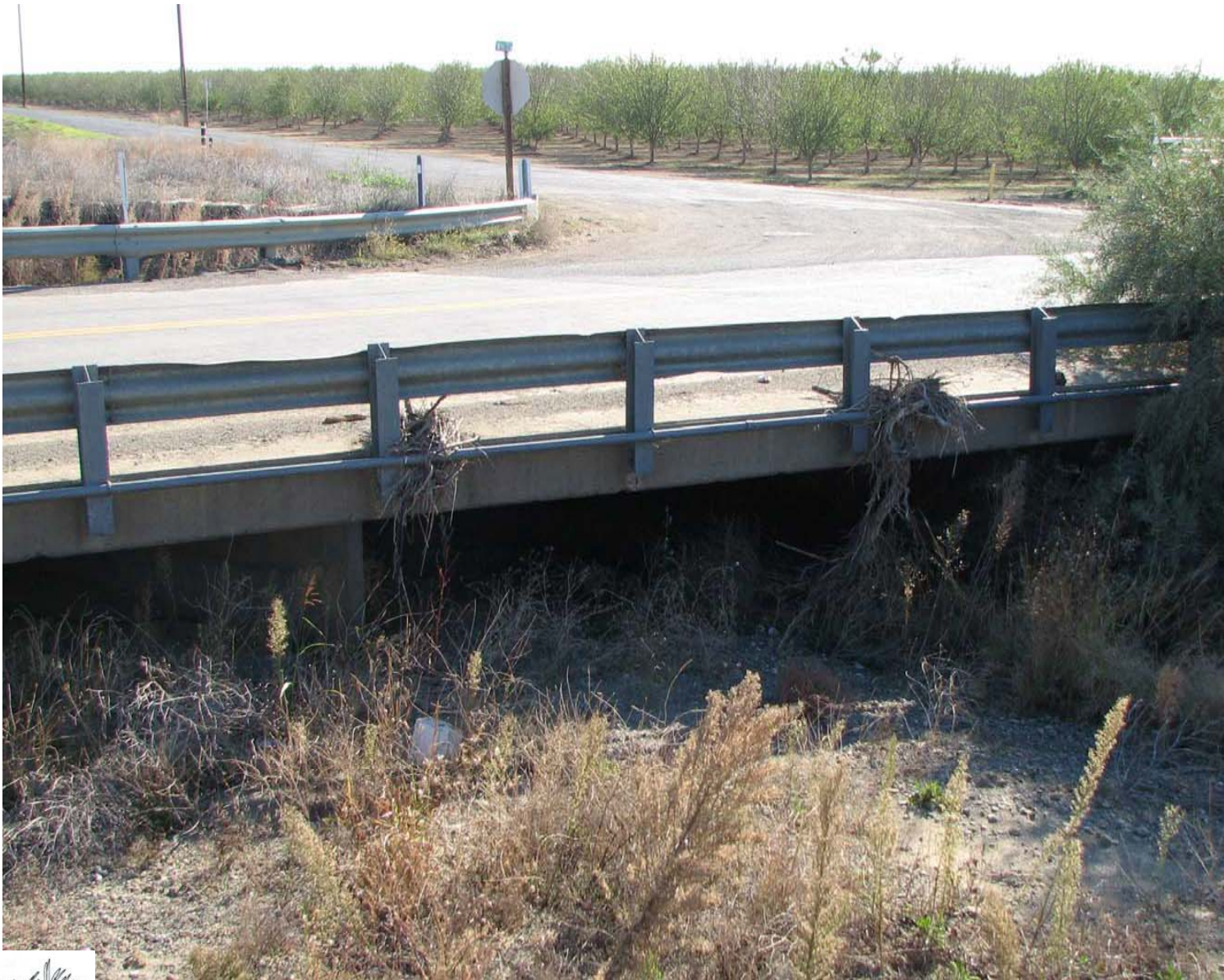
Figure 3-Geomorphology. Photo of Clarks Ditch (Petroleum Creek) looking southeasterly and downstream from left bank to College City Road bridge. The headroom beneath the bridge low chord is only 3-4 ft. The bridge deck is at grade. White Road intersection in background. November 6, 2007.
