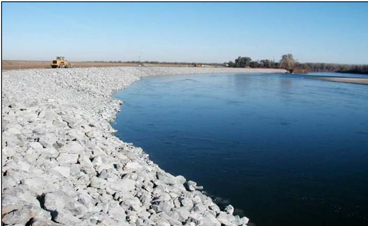
Figure 11. Agency revetment placed on an eroding bank on the middle Sacramento River under Executive Order S-01-06. Photo by Joe Silveira (USFWS), 2007.
