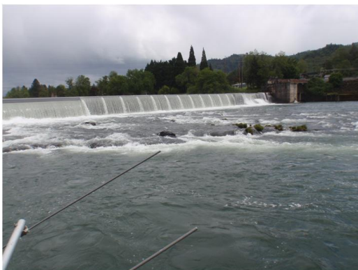
Photo 3: 3/24/2010 (downstream of dam)
