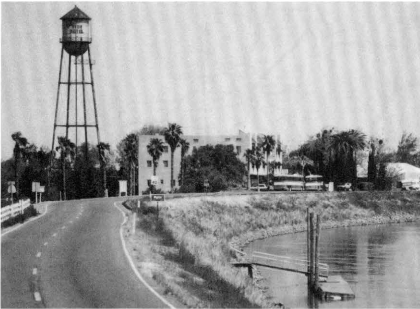
The town of Ryde is one of many communities protected from flooding by project levees.
