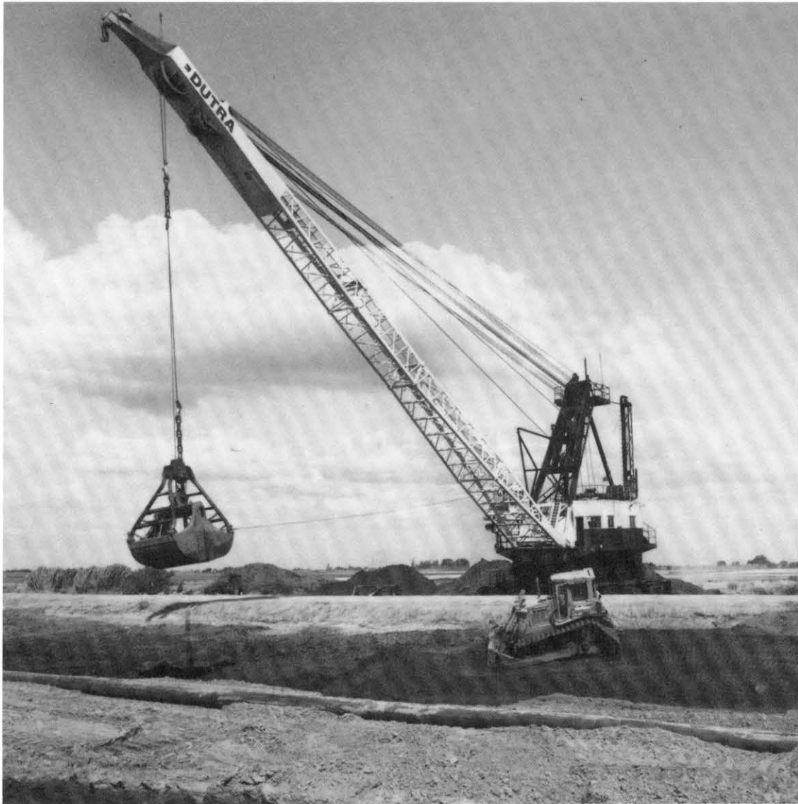
Levee rehabilitation on Twitchell Island.
