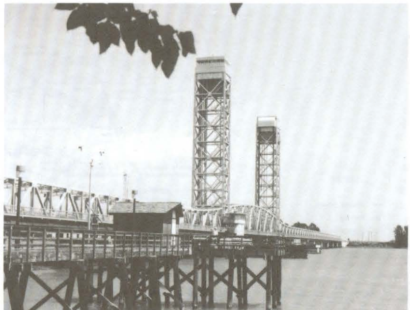
Rio Vista bridge on State Highway 12.
