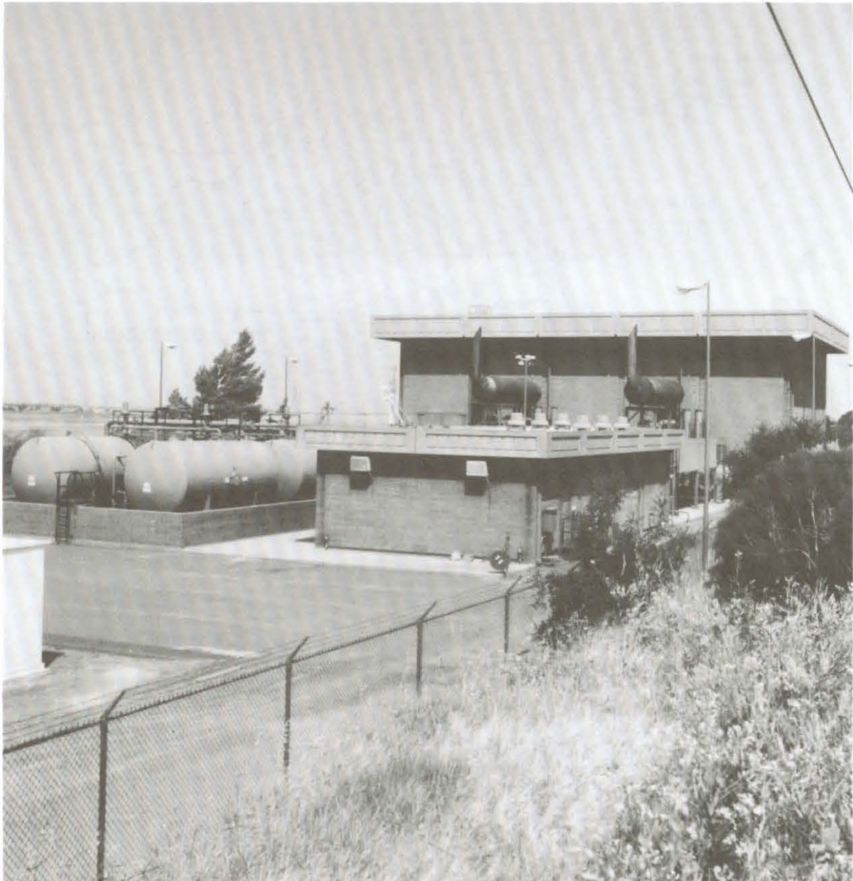
One of Pacific Gas and Electric Company's natural gas facilities on Brannan Island.
