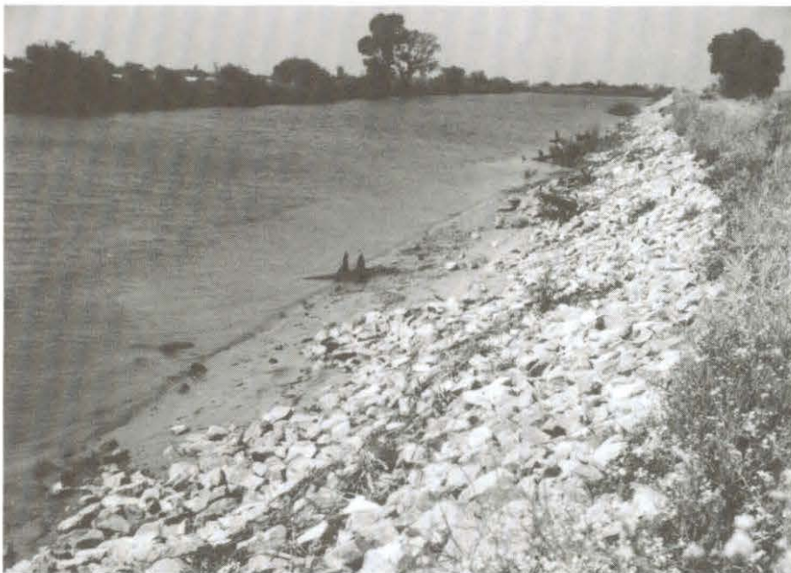
Some levees are protected from erosion by riprap.
