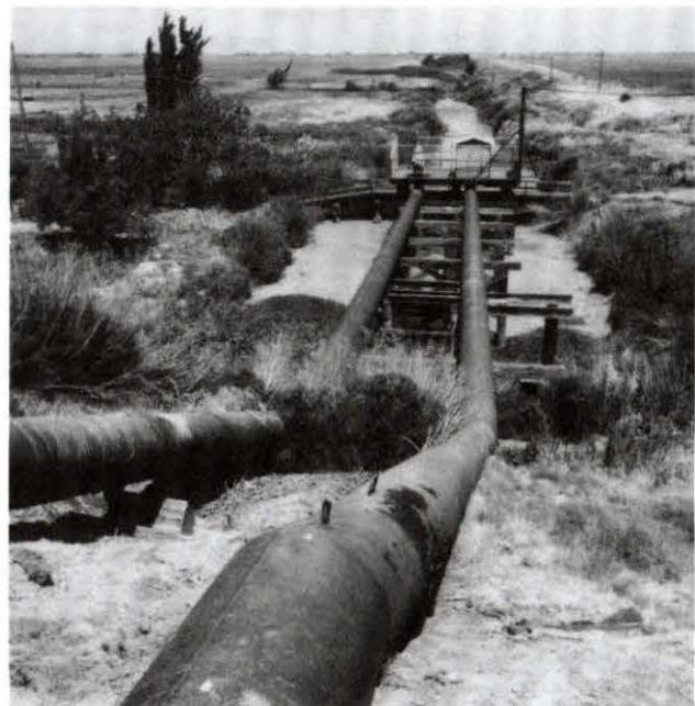
Agricultural drainage pipes on Twitchell Island. (The water is lifted approximately 20 feet to flow into the San Joaquin River.)
