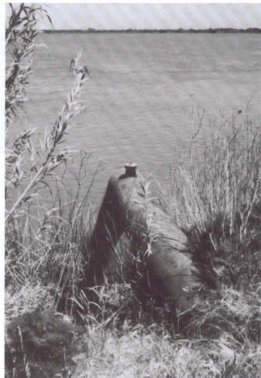
A siphon diverting water from the San Joaquin River to irrigate Sherman Island cropland.
