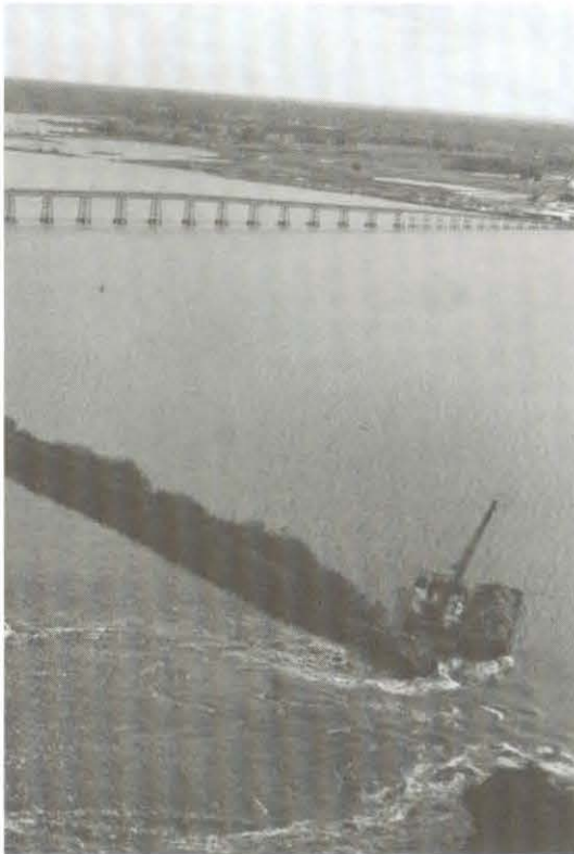
Levee break on Sherman Island in 1969.
