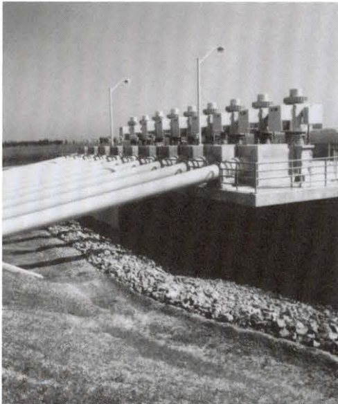
North Bay Aqueduct Pumping Plant at Barker Slough.
