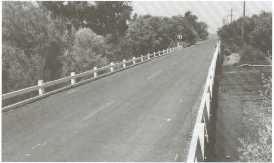
Looking west on Lambert Road crossing Snodgrass Slough west of Courtland.
