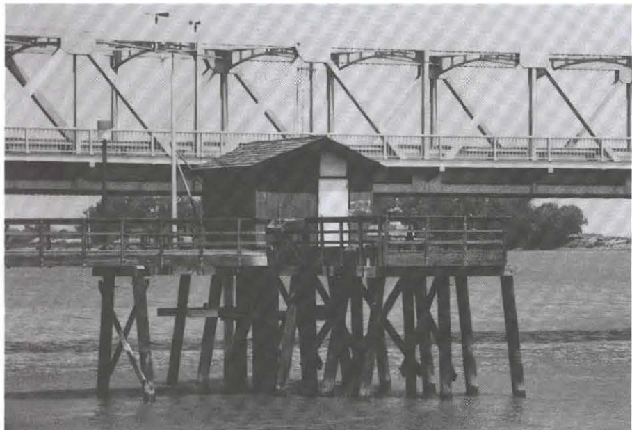
Fixed monitoring station at Rio Vista continuously monitors water level, salinity, temperature, dissolved oxygen, turbidity, and pH. It also measures wind speed and duration and solar radiation. It is one of over 35 stations in the Delta.
