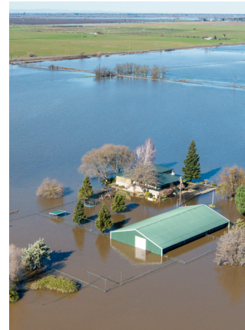
After several years of drought conditions, heavy storms brought unrelenting snow and rain to Central California mountains and valleys during the first two months of 2017, which resulted in significant flooding. Shown in January 2017, these inundated agricultural structures are located outside Elk Grove, south of Sacramento.
