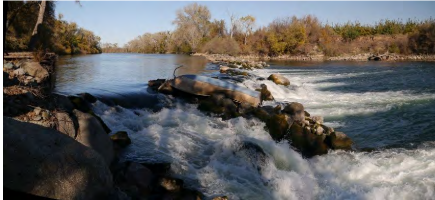
Figure 2-39. The Boulder Weir at Sunset Pumps
