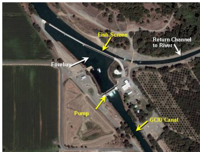
Glenn-Colusa Irrigation District Canal Intake Source: DWR, 2007
