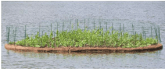
Figure 4.8. Floating wetland islands enhance removal of nutrients, provide habitat for fish and wildlife, and can enhance aesthetics. Photo credit: Cascade Meadow Wetlands and Environmental Science Center, Saint Mary's University, Rochester, Minnesota.
