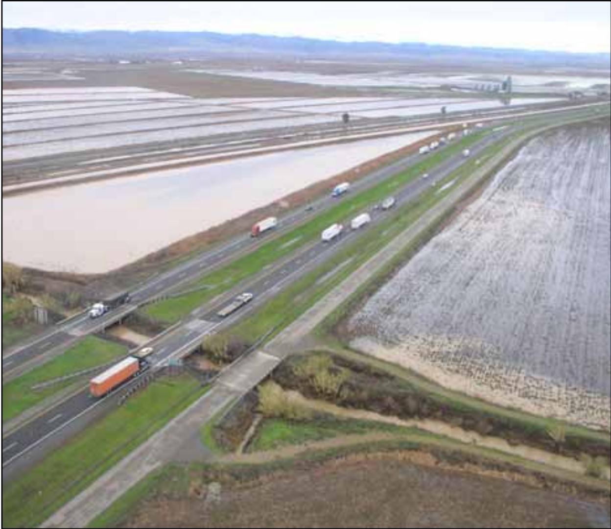
Interstate 5 (Photo: Jack Alderson)
