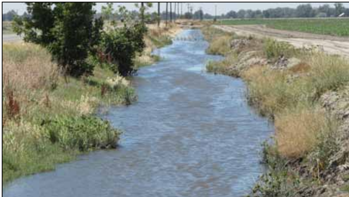
Irrigation ditch (Photo: Mary Fahey)
