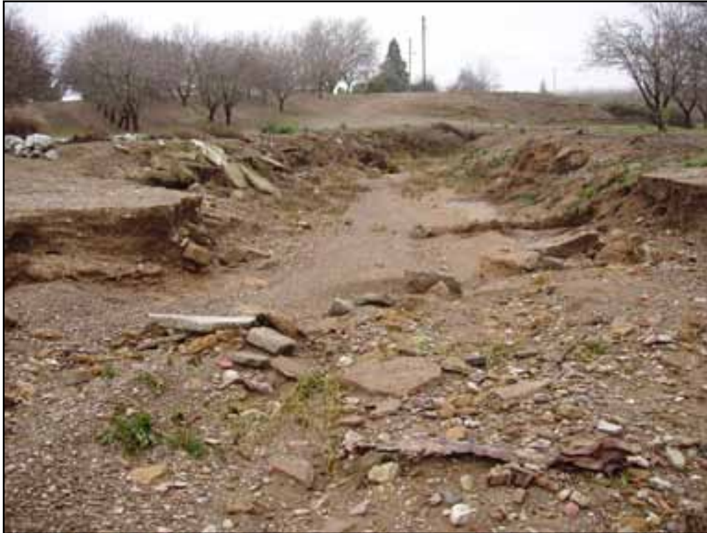
Vegetation along this streambank would help stabilize the banks and filter runoff from the adjacent orchard (Photo: Jennifer Masters)
