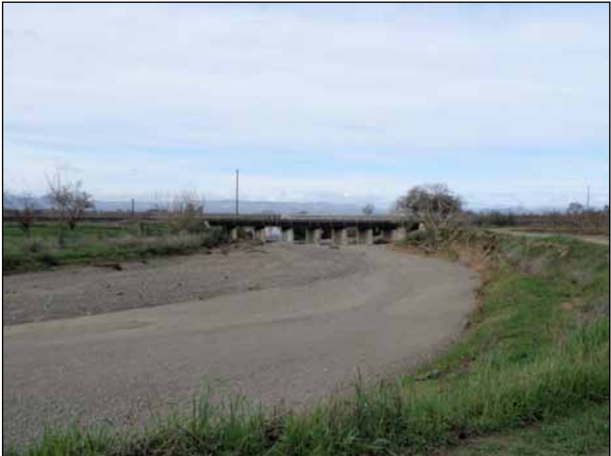
Interstate Highway 5 passes over Buckeye Creek in Yolo County (Photo: Phil Hogan)
