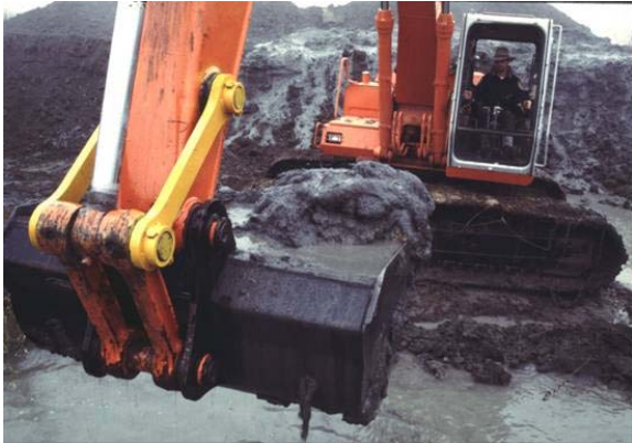
Cleaning out mud from pump station sump
