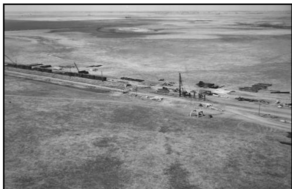
Trestles being rebuilt in 1950s
