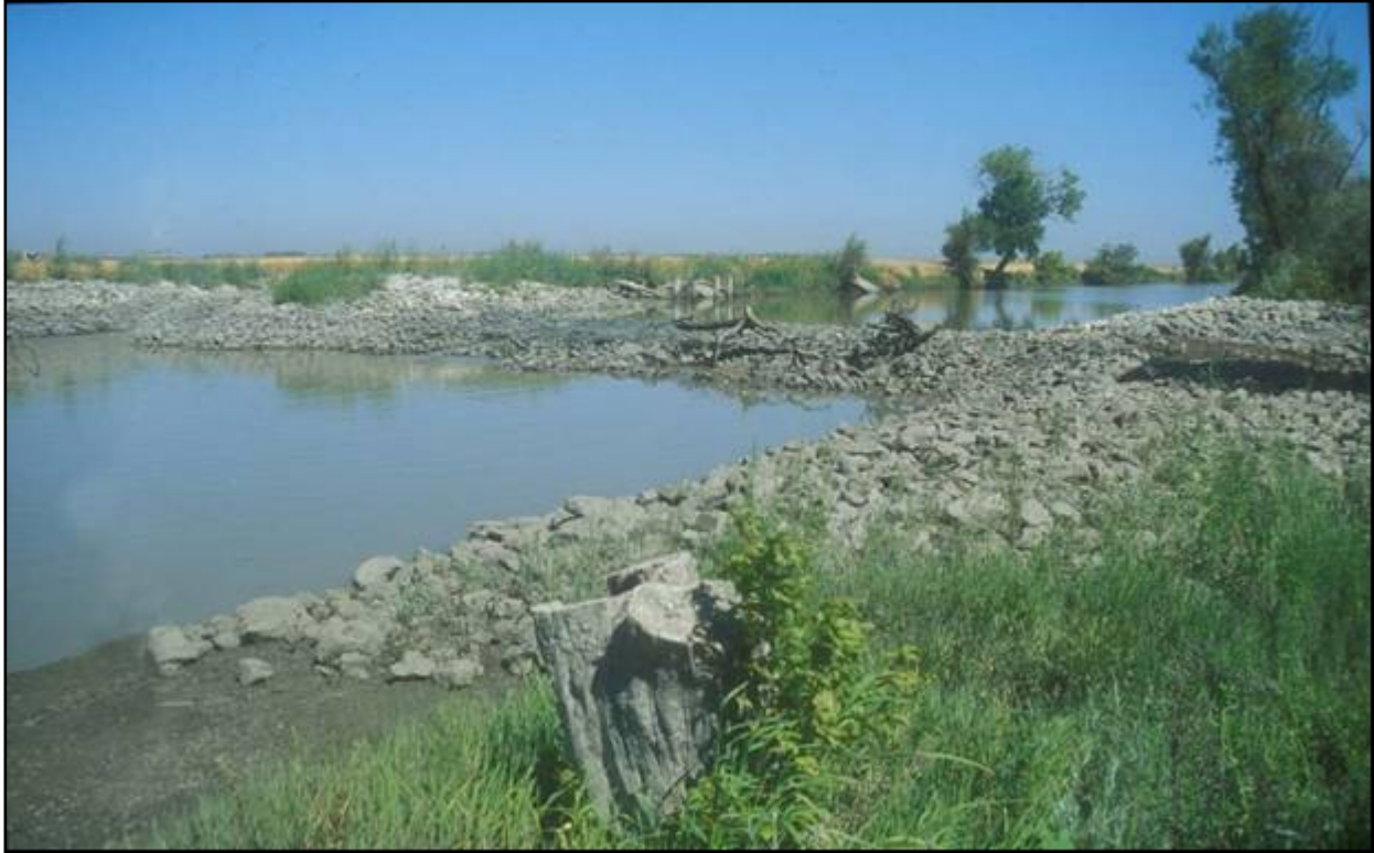
Lisbon Weir, looking north (upstream) the East Toe Drain
