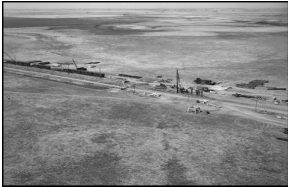
Trestles being rebuilt in 1950s
