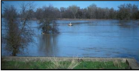
Water flowing over the Fremont Weir
