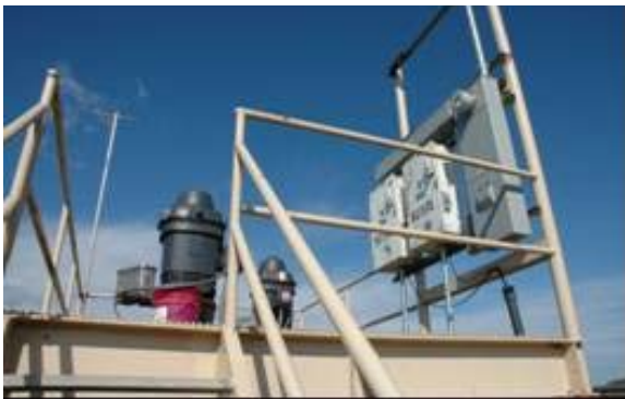
Platform of elevated pump station
