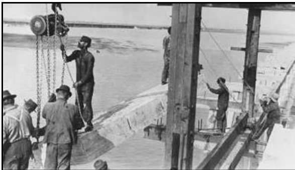
Construction of the Yolo Causeway – 1915
