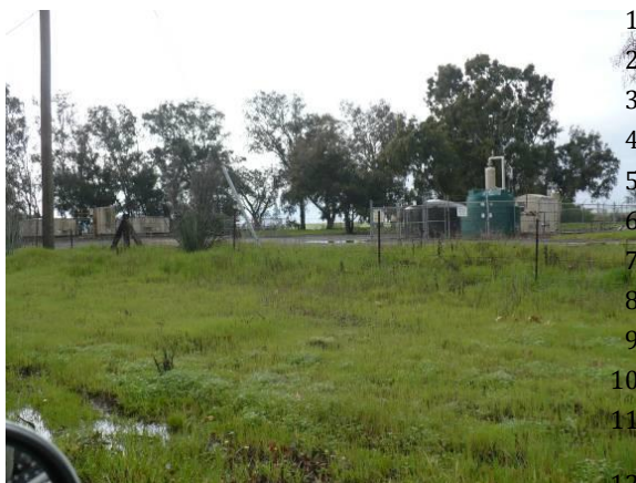
Figure 24A.4-2. Oil and Gas Production
