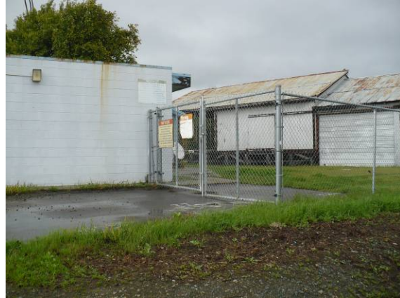
VIEW TOWARD THE: NORTHEAST
