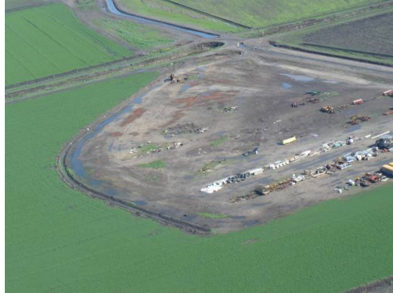
VIEW TOWARD THE: NORTHEAST
