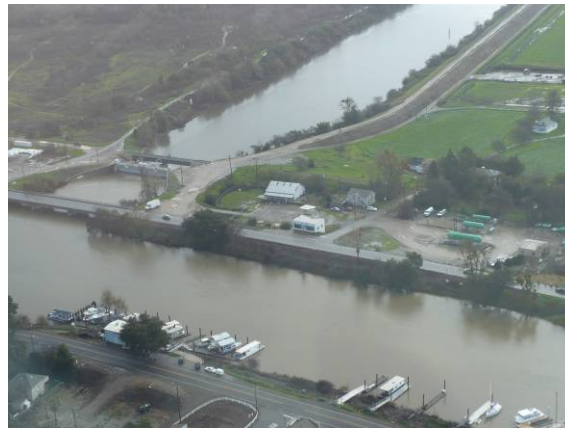
VIEW TOWARD THE: NORTHEAST
