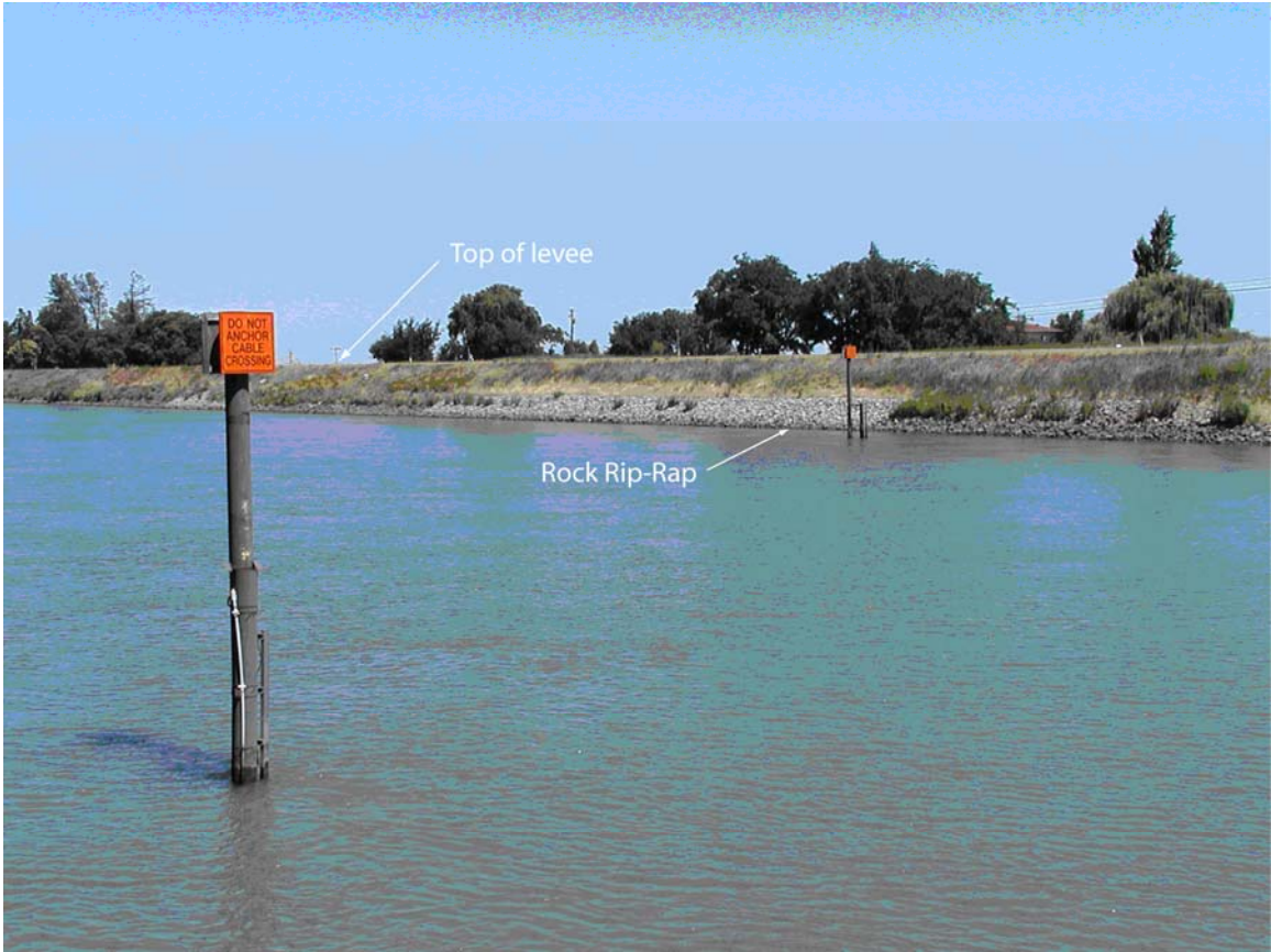
Figure 1.2 – Photograph of the Sacramento River at station WGA. Flow monitoring equipment is mounted on the pilings shown.
