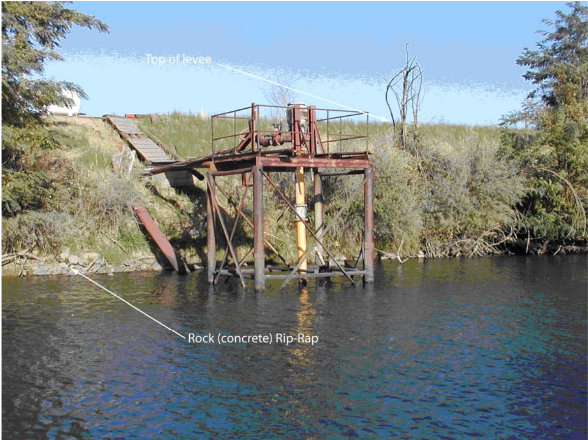
Figure 1.5 – Photograph of the USGS flow station in Sutter Slough. Flow monitoring equipment is mounted on the pump stand shown.
