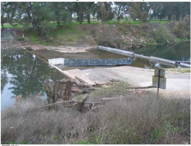
Photo 4-23 Mormon Slough—Bellota Weir with temporary fish ladder
