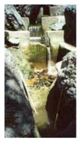
Photo 4-3 Big Chico Creek—Iron Canyon's worn concrete and collapsed floor /DWR photo
