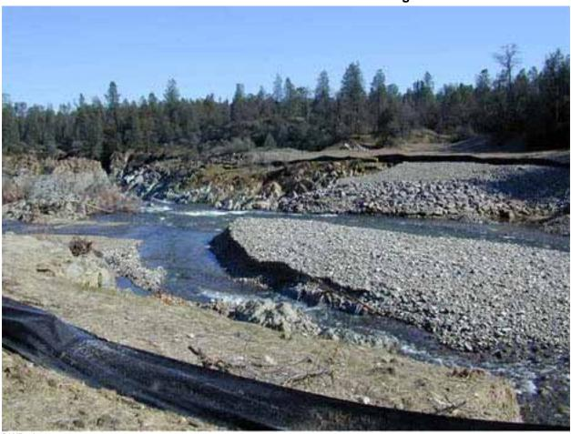
Photo 4-8 Clear Creek after removal of armored gravel berm
