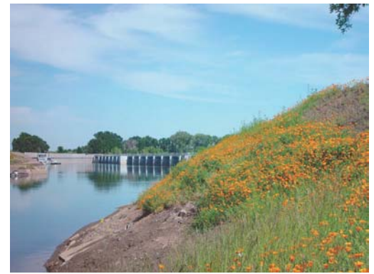
View of poppies in pump station forebay; fish screen in background
