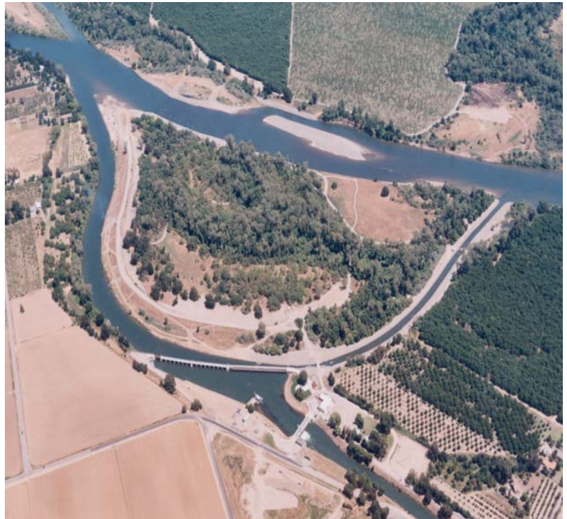
Aerial photo of the District facilities
