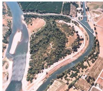
Aerial photo of District facilities, including the gradient facility, looking south
