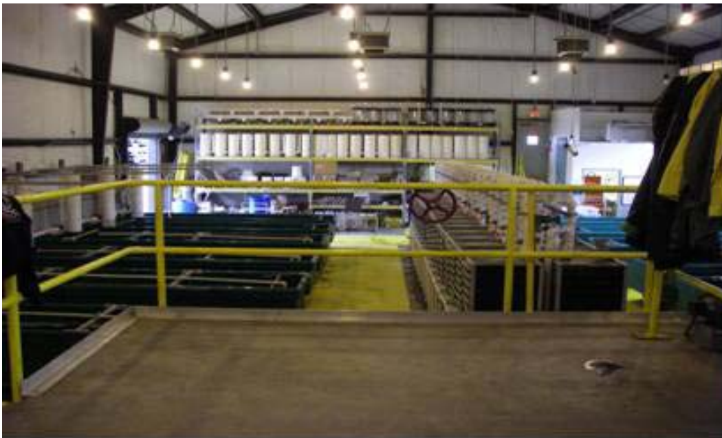
Figure 4-13. Interior of NFH Building 2.
