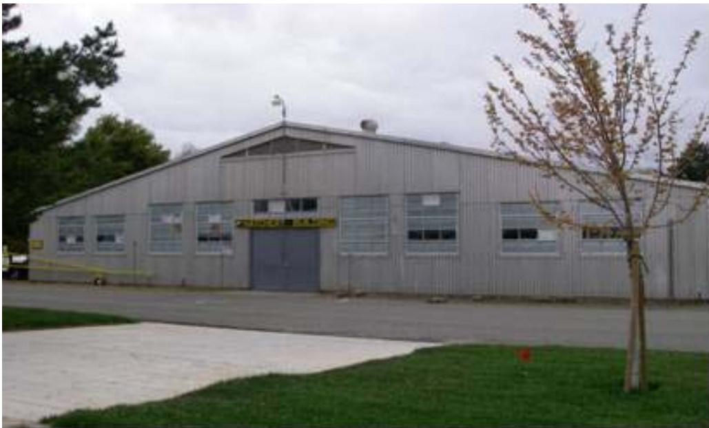
Figure 4-17. Exterior of NFH Building 1.
