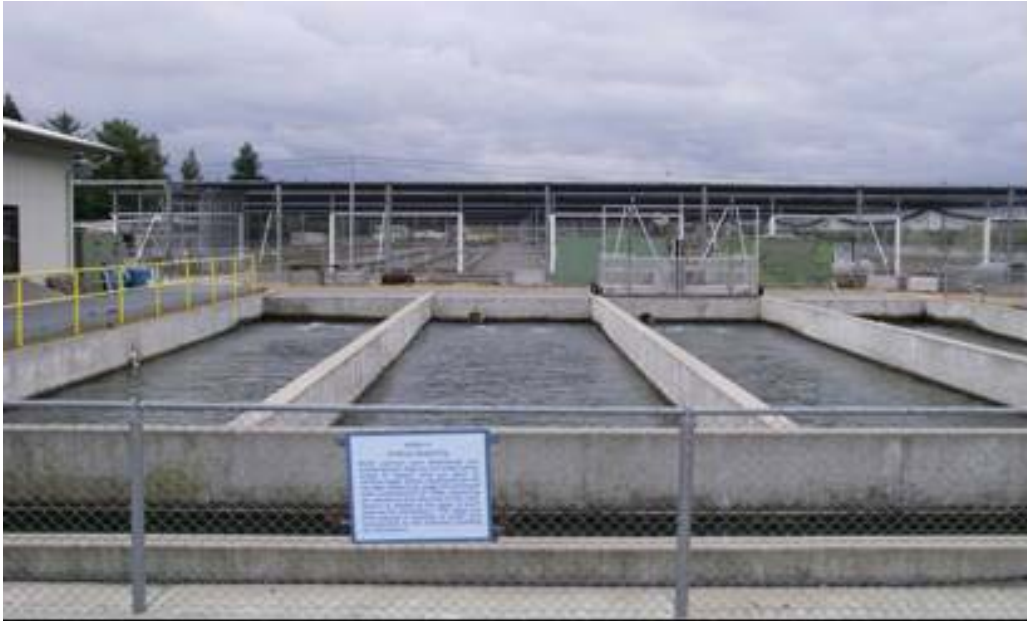
Figure 4-8. Concrete holding ponds adjacent to NFH Building 2 facing west.
