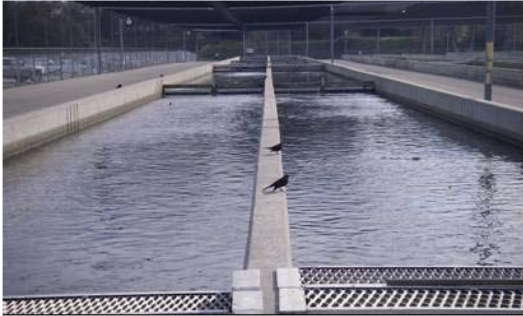
Figure 4-20. Concrete raceway ponds facing north.
