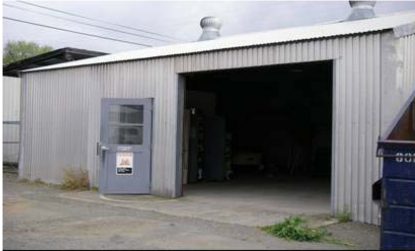
Figure 4-31. Equipment, Paint, and Fuel Storage Building.
