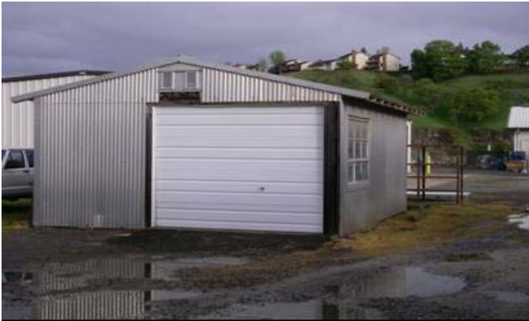
Figure 4-29. Lawn Equipment Building.
