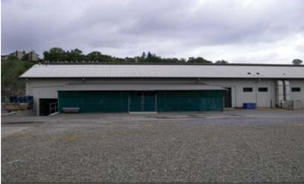
Figure 4-12. Exterior of NFH Building 2.
