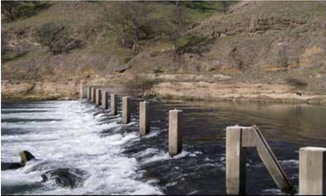
Figure 4-3. Concrete supporting piers in the river facing north on the left bank.
