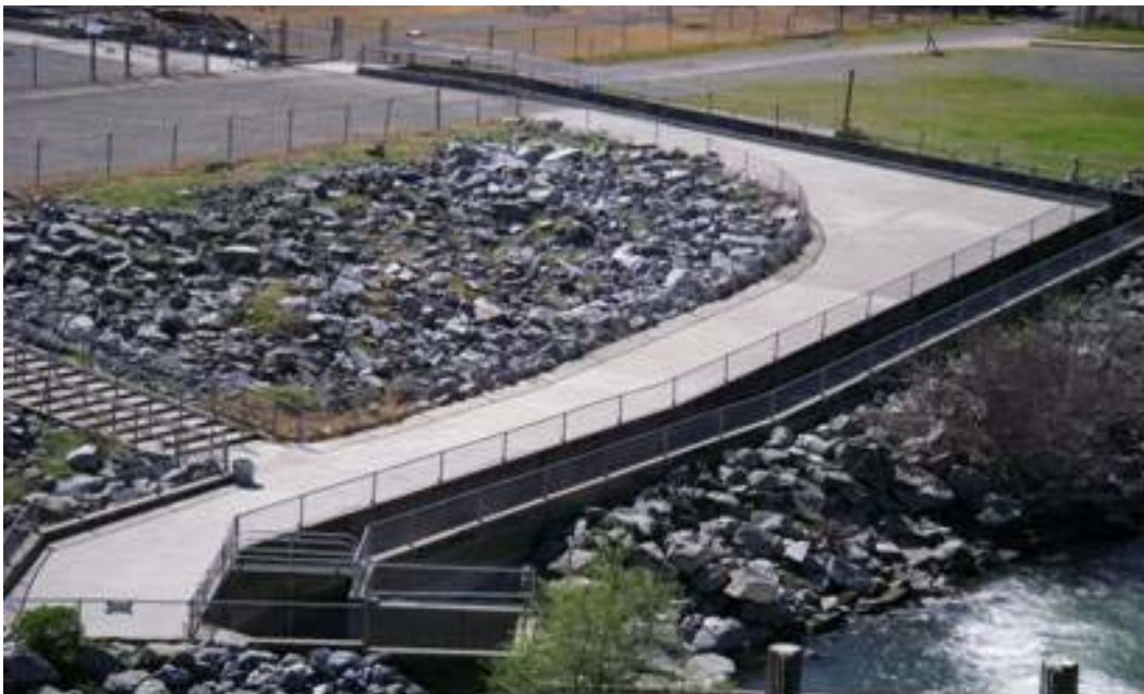
Figure 4-5. Bottom of the fish ladder on the left bank facing west.
