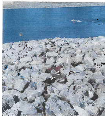
Sheetpile wall with rock slope protection in place
