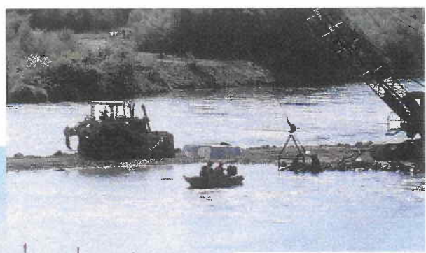
In-river construction using drag line
