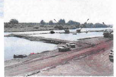
In-river construction using longitudinal berm
