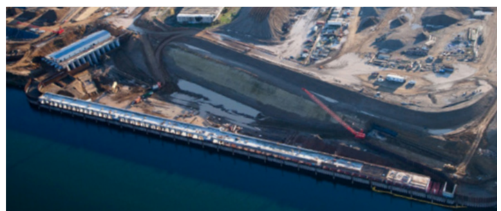
Overview of Fish Screen and Forebay Construction (November 2011)
