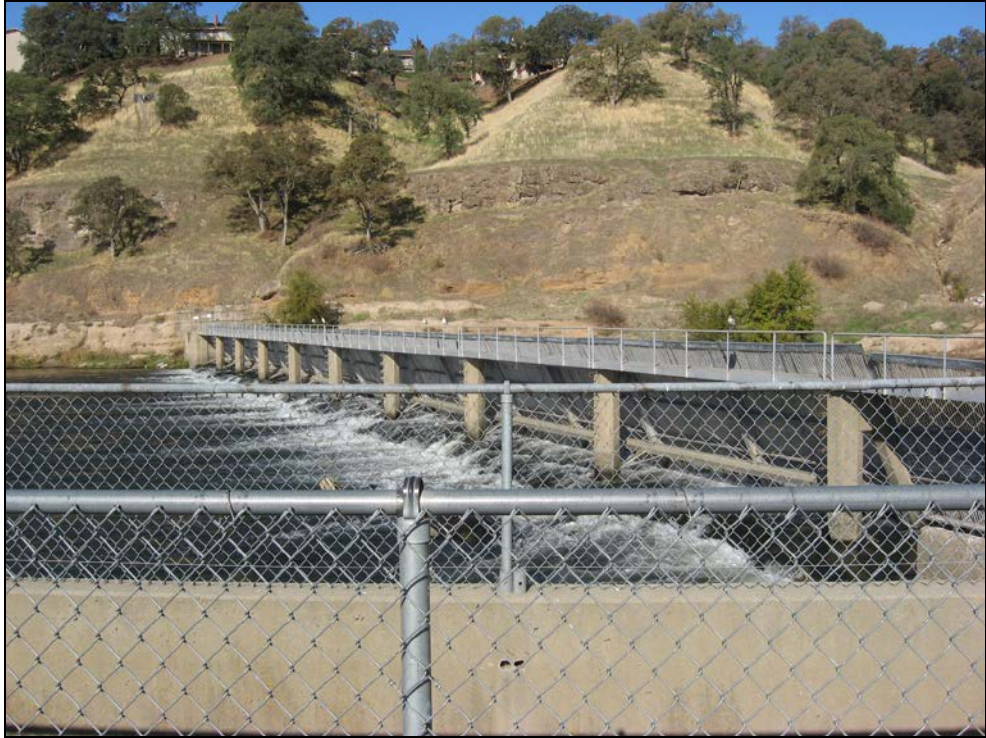
Figure 2-1. Existing diversion weir with superstructure
