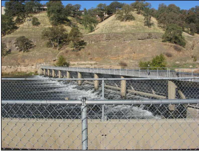
Figure 3-7: Nimbus Weir with superstructure in place
