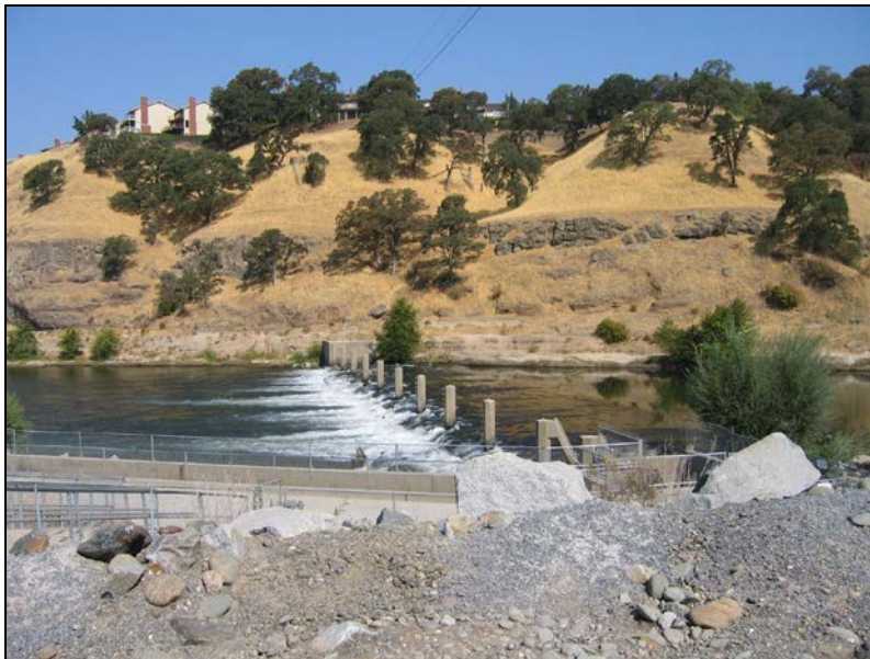
Figure 3-8: Nimbus Weir with superstructure removed (Note concrete piers)
