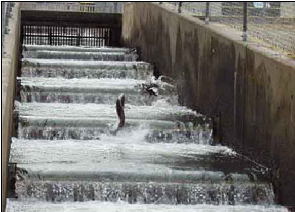
Figure 2-2. Existing fish ladder
