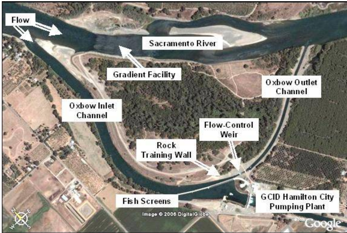
Figure 2. The GCID Hamilton City Pumping Plant and associated features of the Fish Screen Improvement Project.
