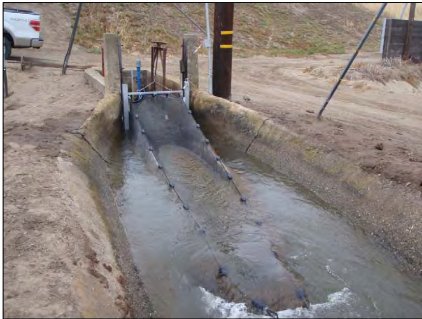
Figure 13. The fyke net and associated apparatus used to sample for fish entrainment in the Cranmore trapezoidal concrete canal.
