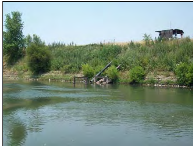
Appendix Figure 23. The South Steiner pump station intakes looking in a downstream direction.
