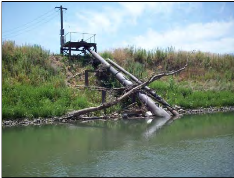
Appendix Figure 37. The Windswept pump station intake looking in a downstream direction\.
