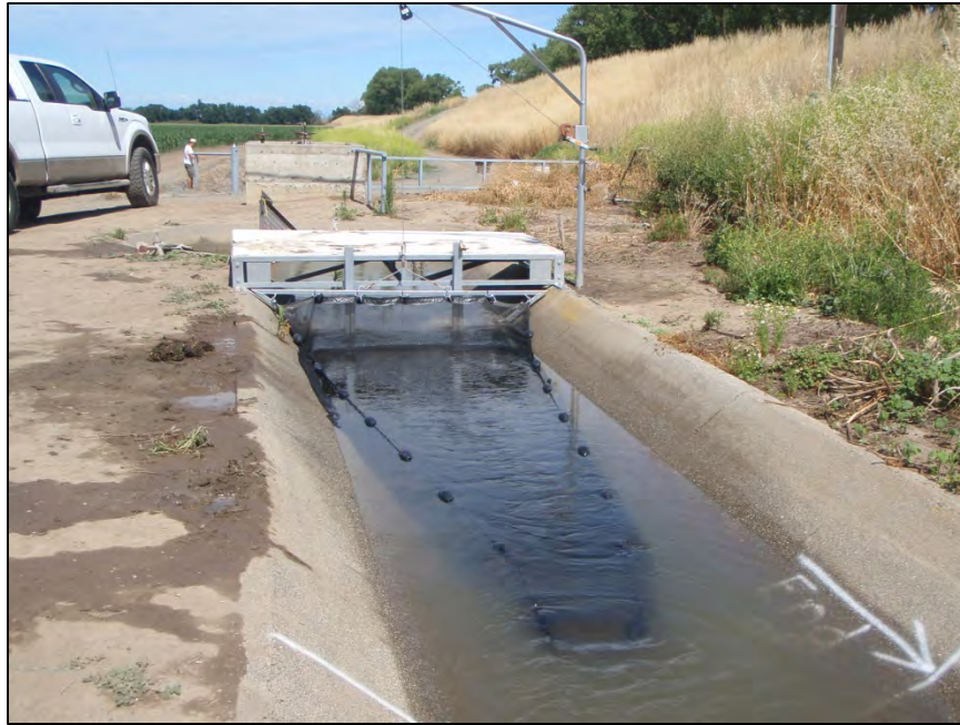
Figure 6. Fyke apparatus and sampling platform used for fish entrainment sampling in the South Steiner concrete canal.
