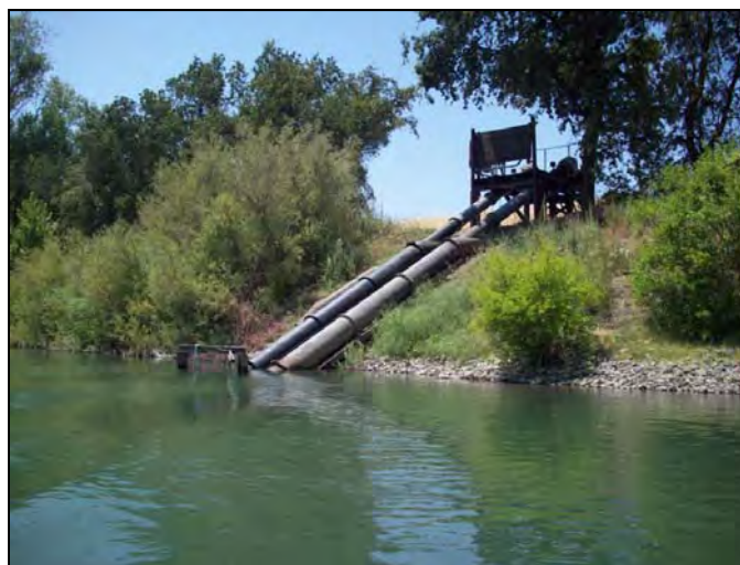
Appendix Figure 2. The Sycamore pump intakes looking in a downstream direction.
