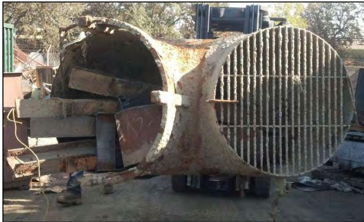
Figure 120. Trash racks (bars) on the Alamo diversion intake pipe shown on its side. Picture was taken after removal from the river prior to installation of an ISI fish screen. Note the individual's boot at the lower left portion of the picture for size reference. Prior to removal, this intake was positioned upwards such that the intake opening and trash racks were horizontal and the river flow went over the top of the intake opening. Photo by ISI.
