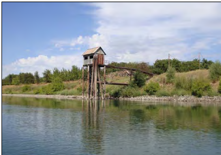
Appendix Figure 65. The Tisdale pump intakes looking in an upstream direction.
