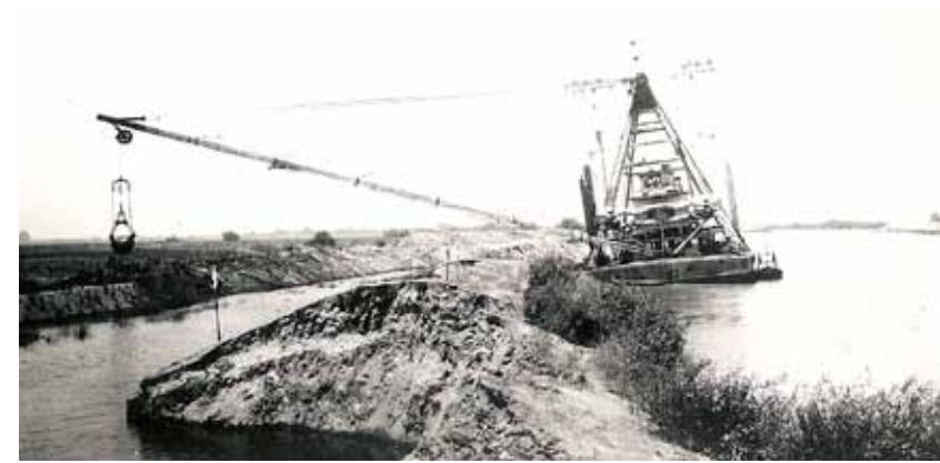
Figure 4.14. Dredge building levee showing side-ditch. This early 1900s photograph shows a sidedraft clamshell dredge working on a levee, drawing material from a ditch. Over the past century, many of these ditches have become a part of the main channel. (Covello ca. 1900, courtesy of Bank of Stockton Historical Photograph Collection)
