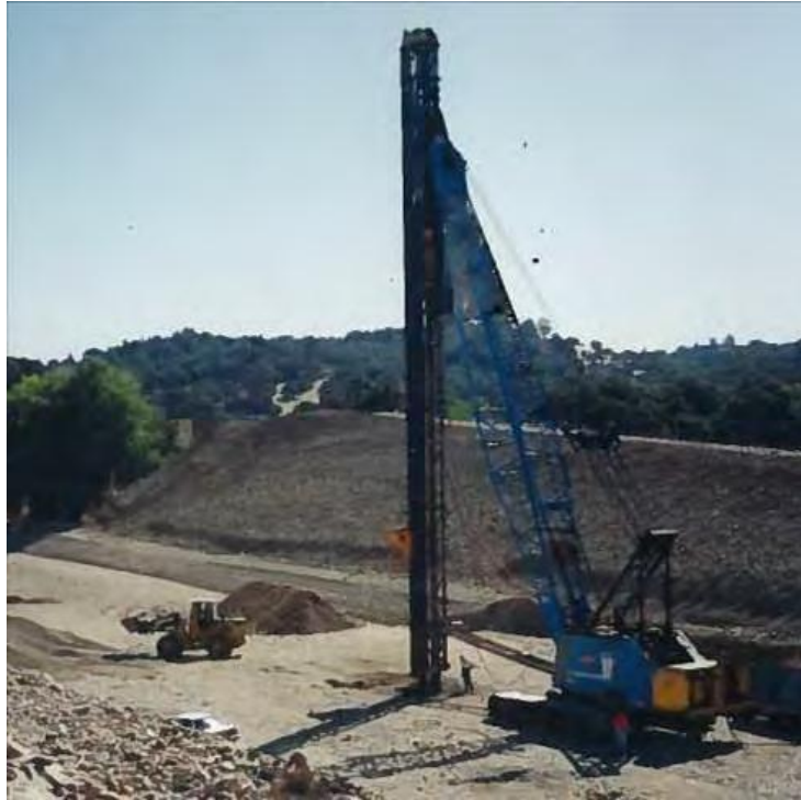
Figure G8. Bottom feed stone column equipment at MIAD in Folsom, California.
