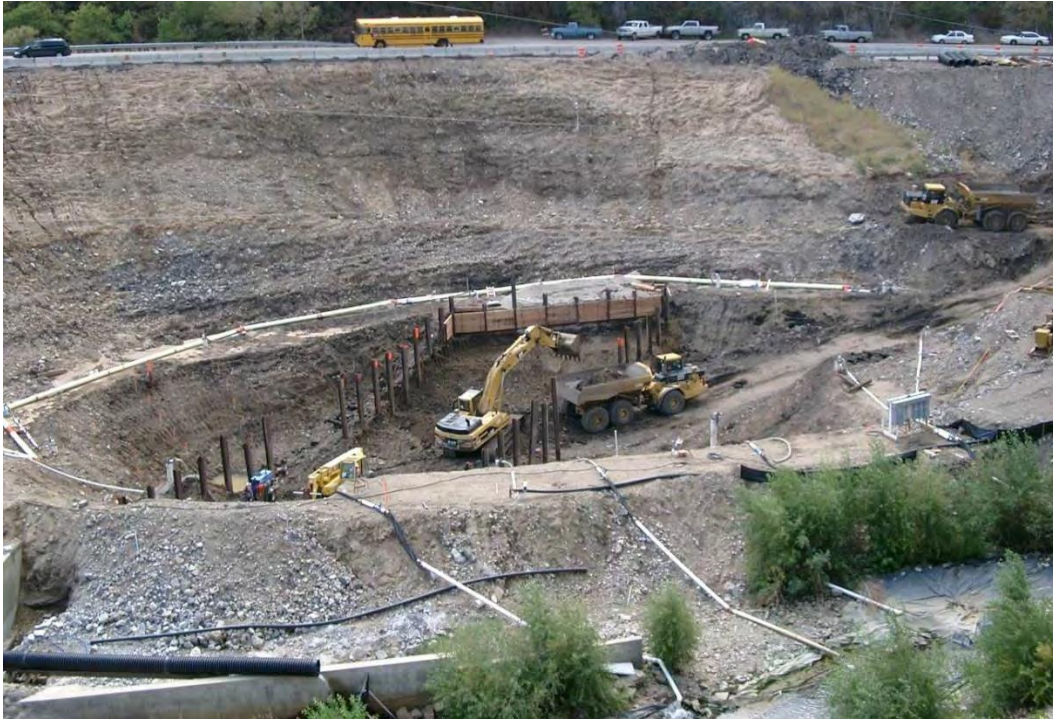
Figure G5. Pineview Dam excavation, dewatering bench, soldier piles, and lagging (2003).
