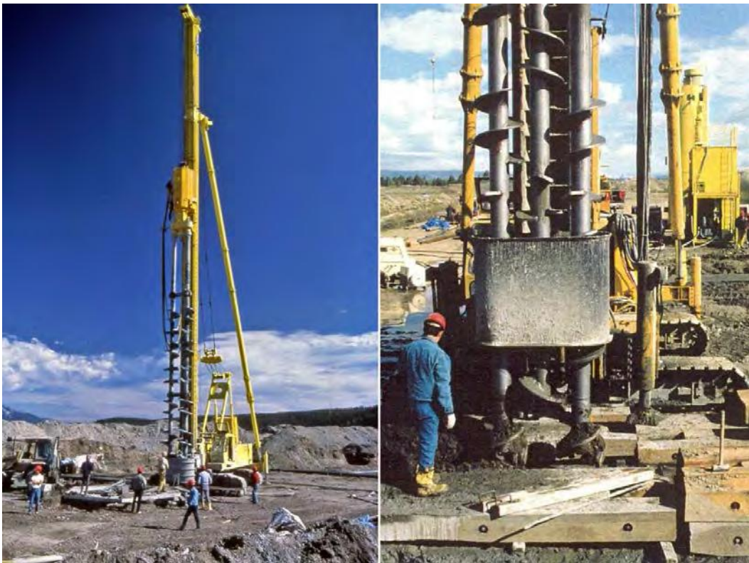
Figure G4. DSM wall construction, Jackson Lake Dam, Wyoming.
