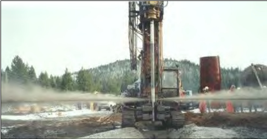
Figure G11. Jet-grout blocks in the foundation of Wickiup Dam.
