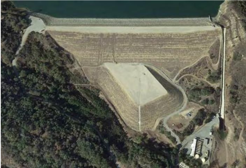
Figure G17a. Casitas Dam stability berm and widened crest.
