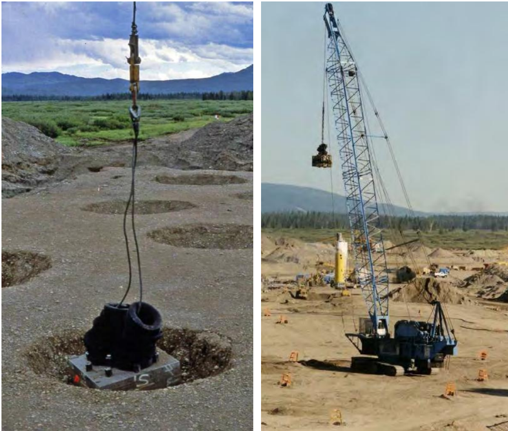
Figure G6a and G6b. Dynamic compaction at Jackson Lake Dam.
