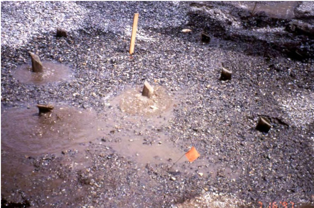
Figure G2b. Layout of stone columns and wick drains for treatment of Salmon Lake Dam foundation, Washington.
