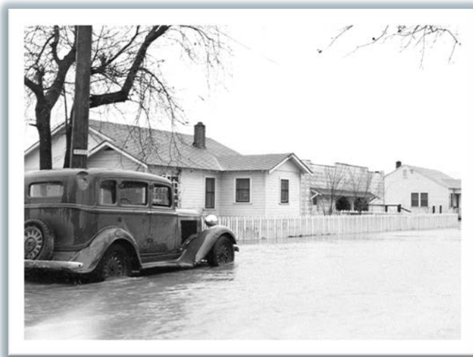
Flooding (2-27-40) in Redding prior to completion of Shasta Dam
