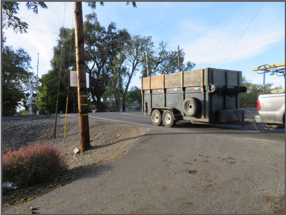
Figure 4.20: Unsafe conditions at an intersection in the City of Tehama due to proximity of RR tracks, lack of shoulders, ditches at sides of roadways.
