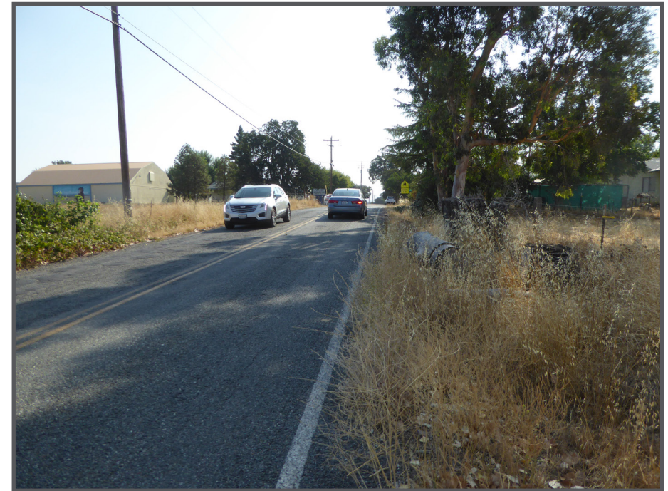
Figure 4.14: Speeding vehicles and lack of shoulders leave no room for pedestrians and cyclists.
