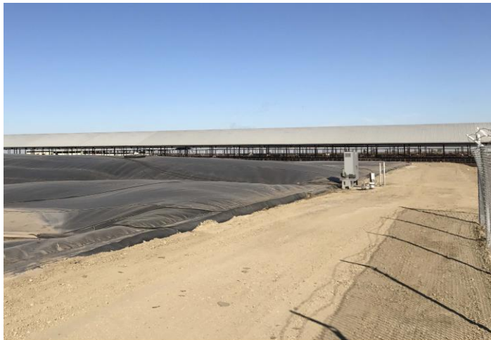
Covered dairy digester lagoon
