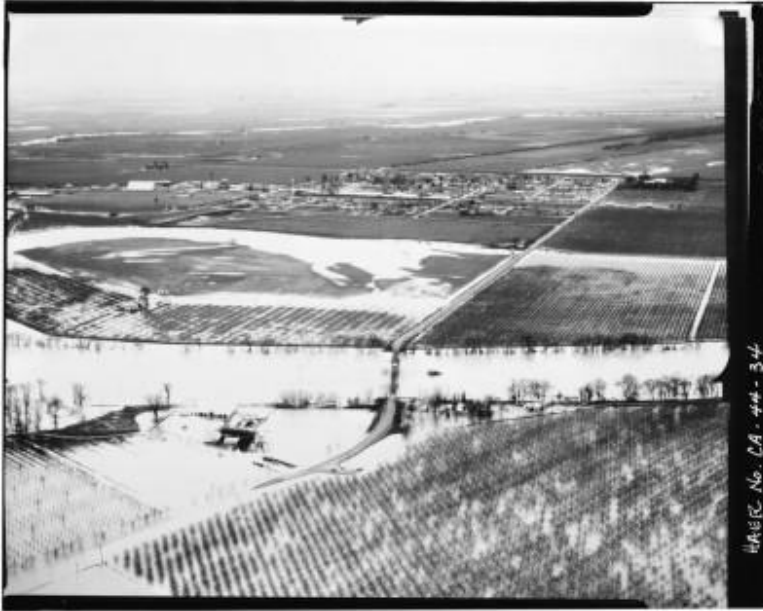
Gianella Bridge Flood of January 24, 1970
