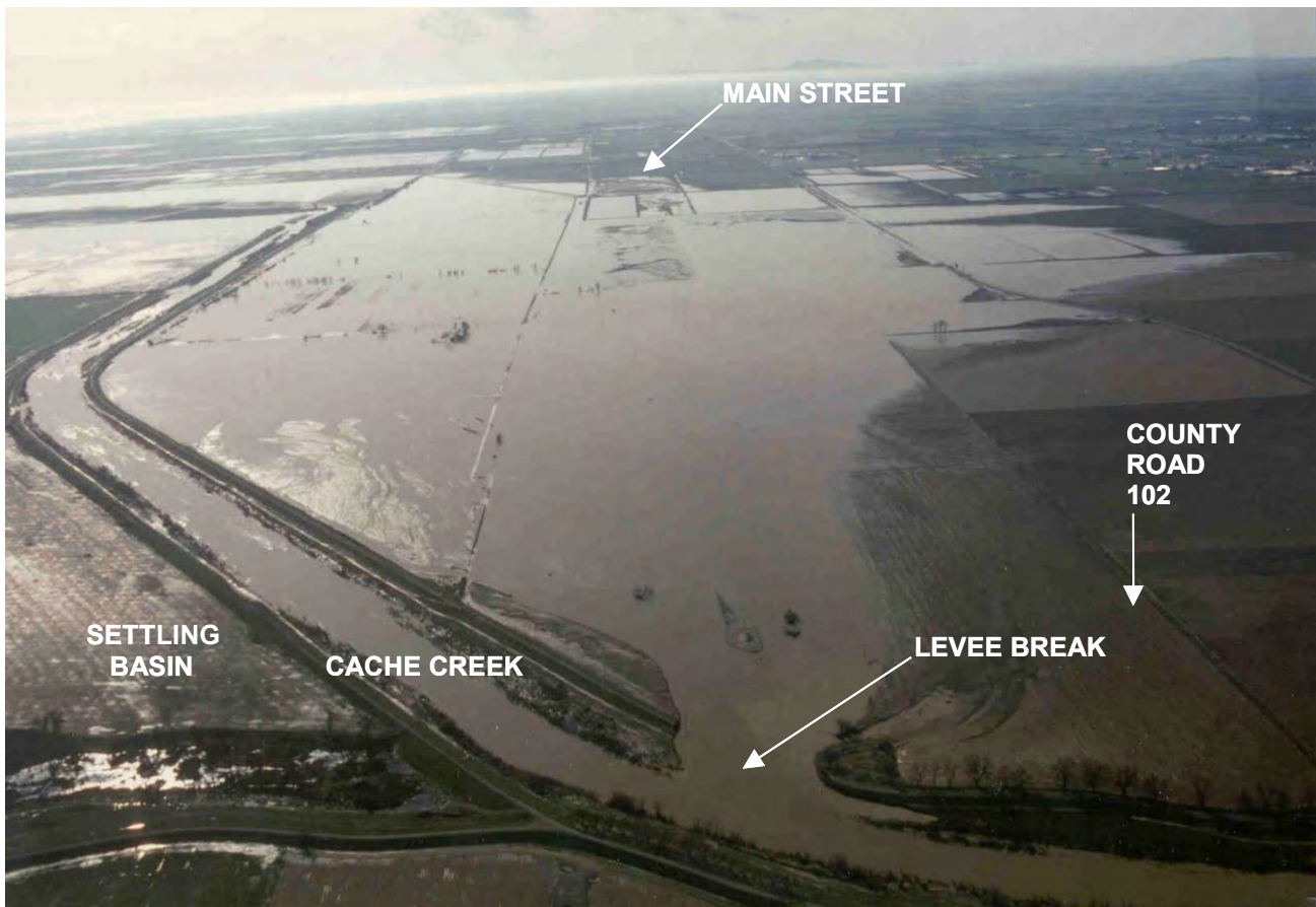
Cache Creek Levee Failure, January 27, 1983, looking south towards Woodland.
