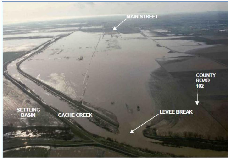
Figure 1: Flooding from Cache Creek in 1983 3
