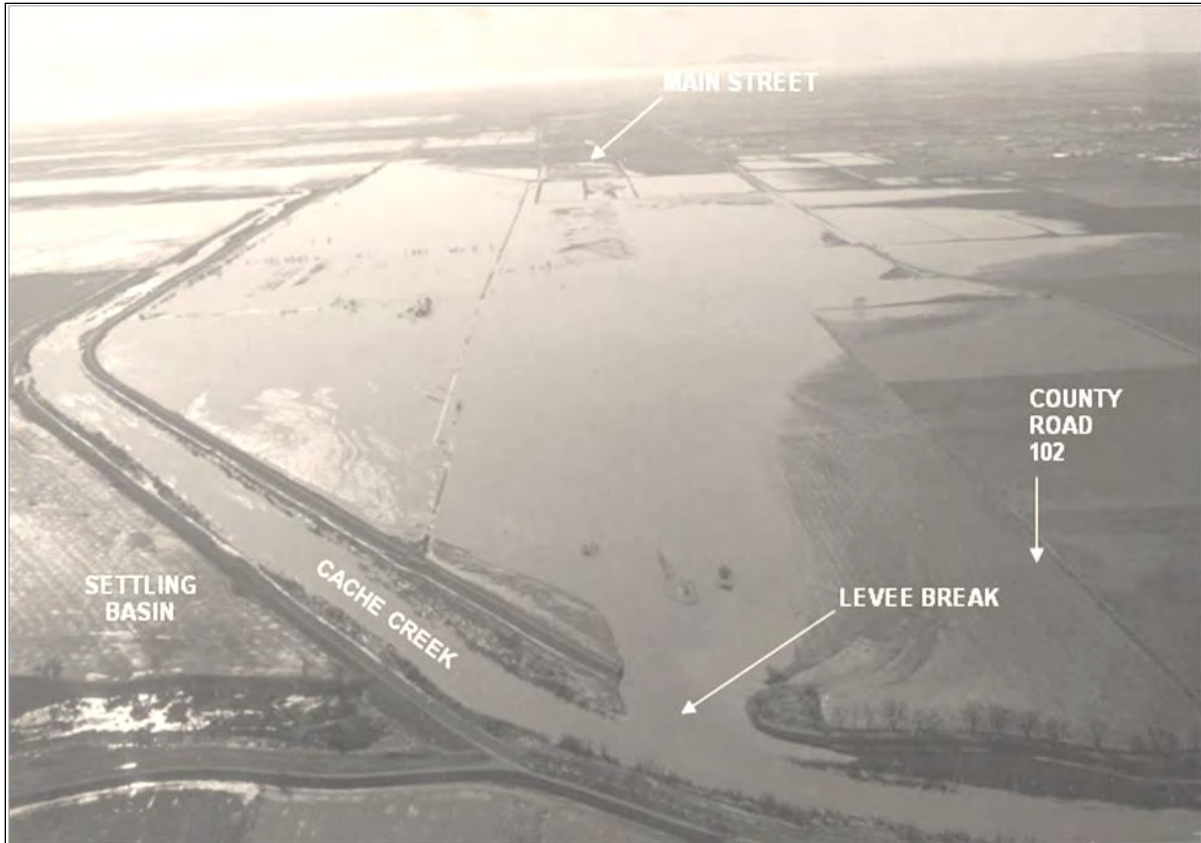
Figure 2-6. Cache Creek Levee Break, 1983
