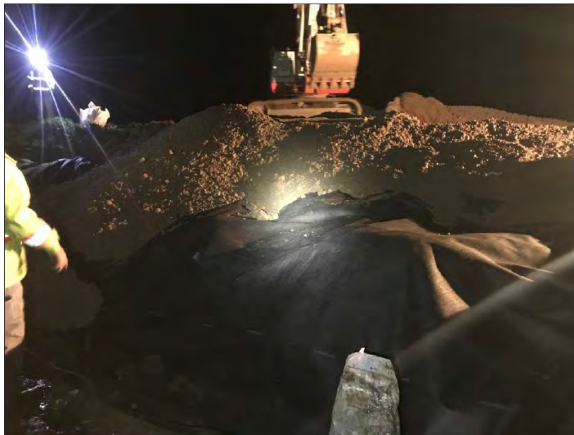
Figure 2-7. Flood Fight Along Existing Cache Creek Levees East of I-5, February 2019
