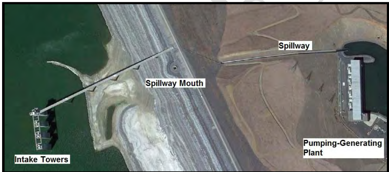
Figure 5. Overview of B.F. Sisk inlet and outlet structures
