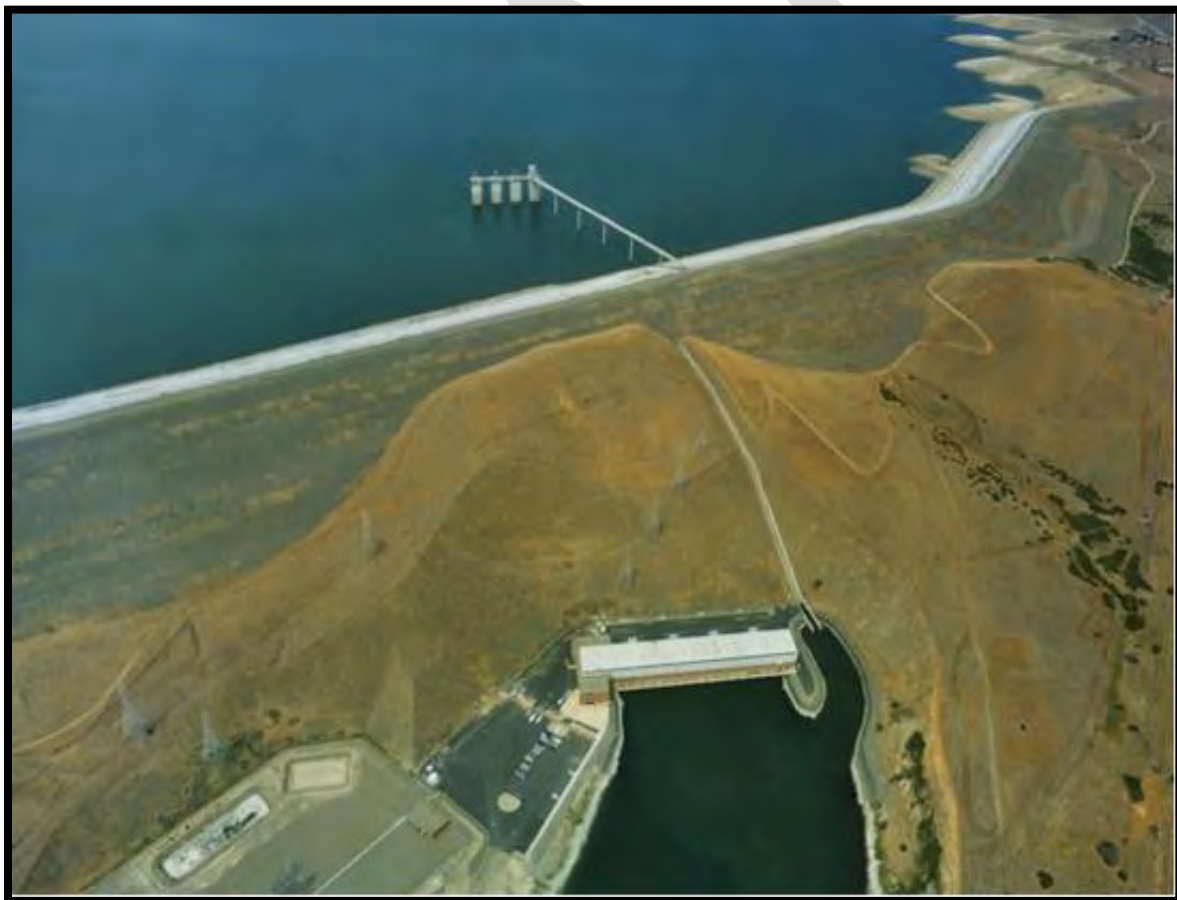
Figure 3. Close-up of B.F. Sisk Dam and Gianelli Pumping-Generating Plant
