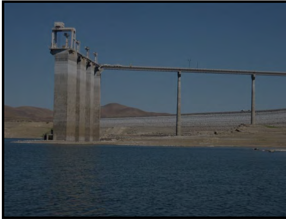
Figure 4. Outlet works intake towers and access bridge
