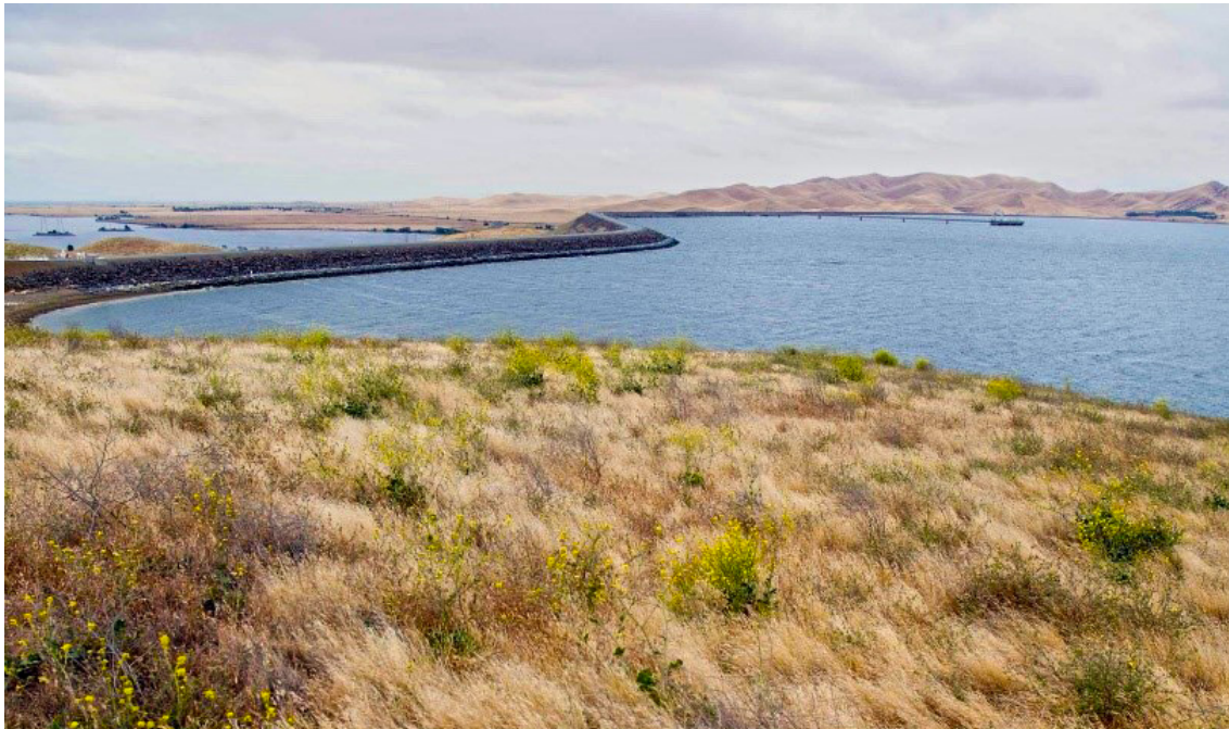
B.F. Sisk Dam and San Luis Reservoir
