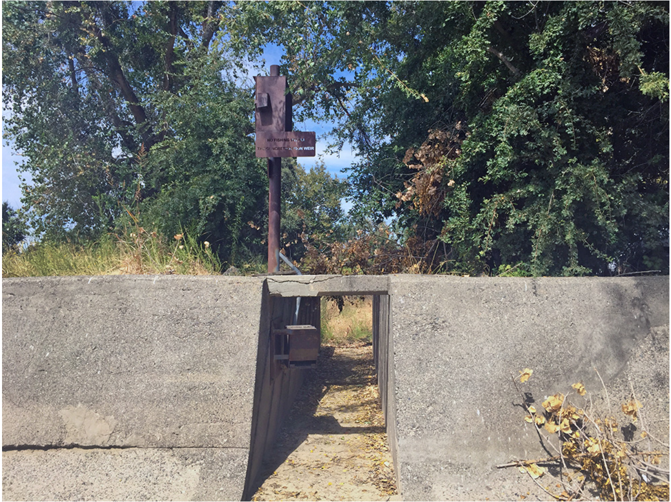
Figure 1 - Fremont Weir fish ladder installed in 1965
