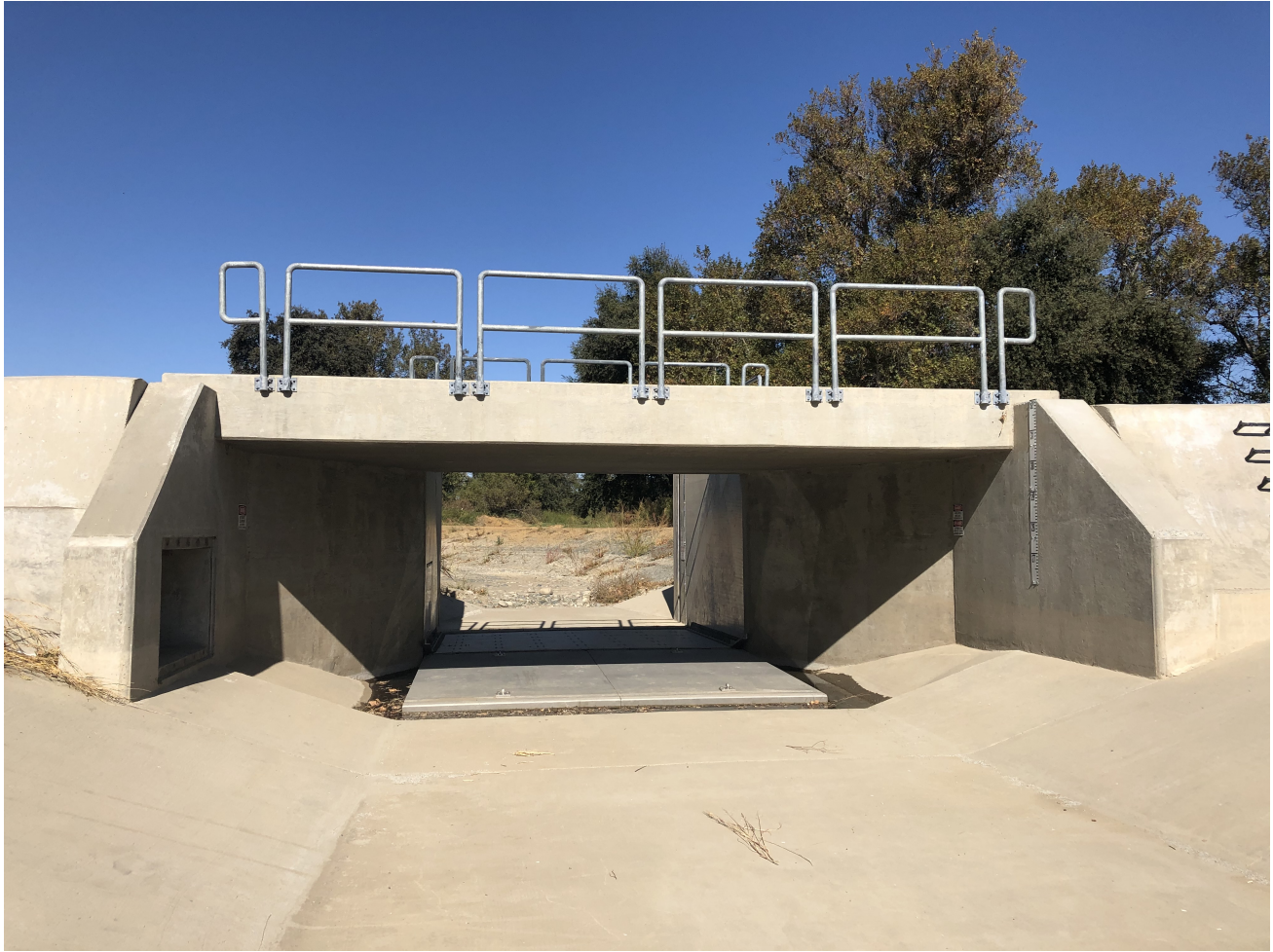
Figure 2 - Fremont Weir fish ladder replaced in 2018
