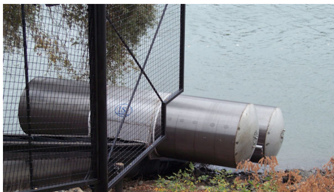
RD 999 Retractable Fish Screen on the Sacramento River. (Photo courtesy of Family Water Alliance)
