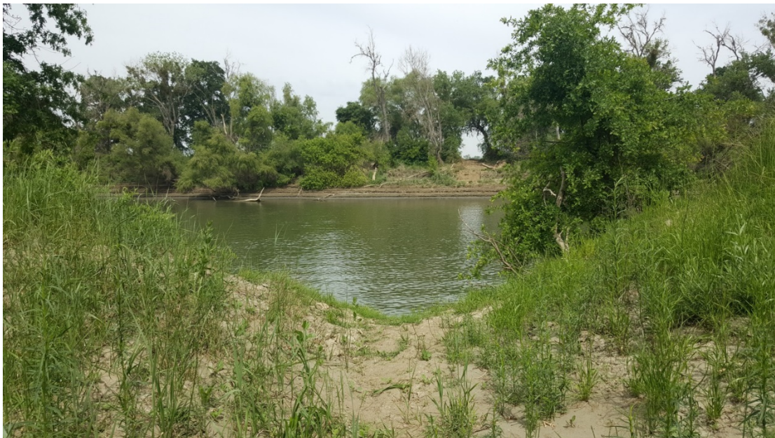
Figure 14-4. Fremont Weir fish ladder intake channel – photo taken at the end of the intake channel looking north at the Sacramento River (May 2016).
