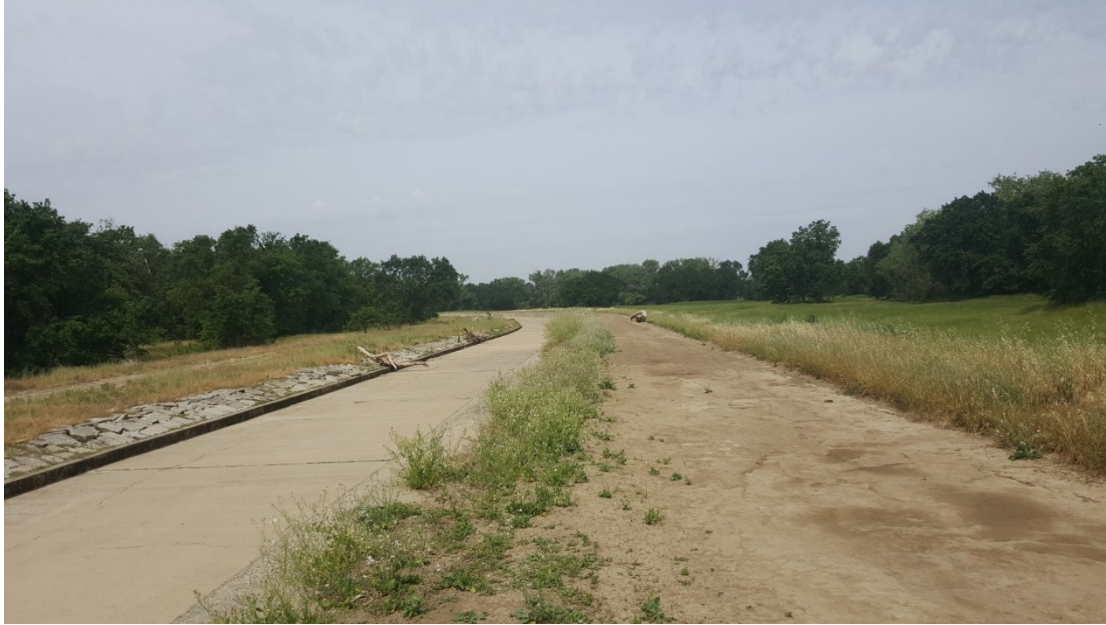
Figure 14-3. East Fremont Weir Headworks location – looking west along the weir crest (May 2016).
