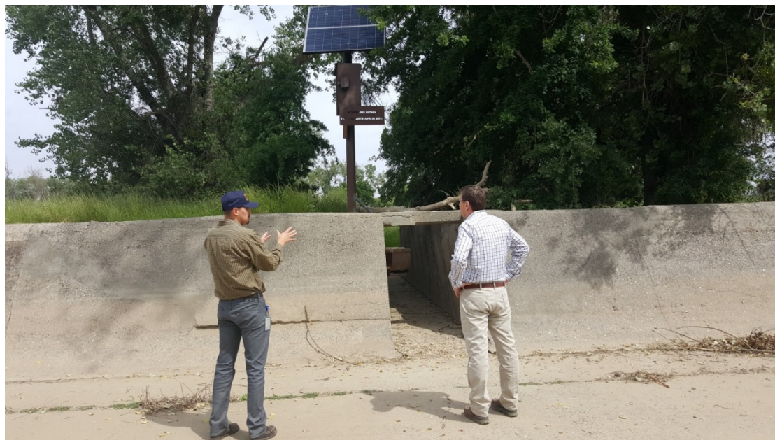
Figure 14-7. Fremont Weir fish ladder intake channel – photo taken from the bypass side of Fremont Weir looking north at the face of the weir (May 2016).
