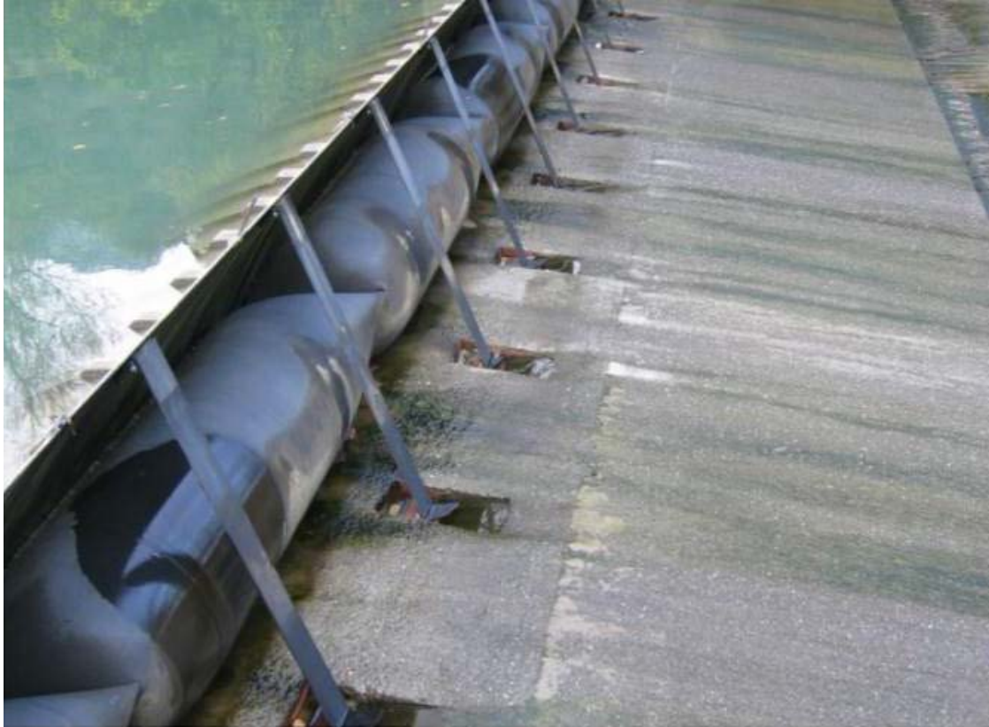
Figure 4-15. Example of Obermeyer-Style Inflatable Gates
