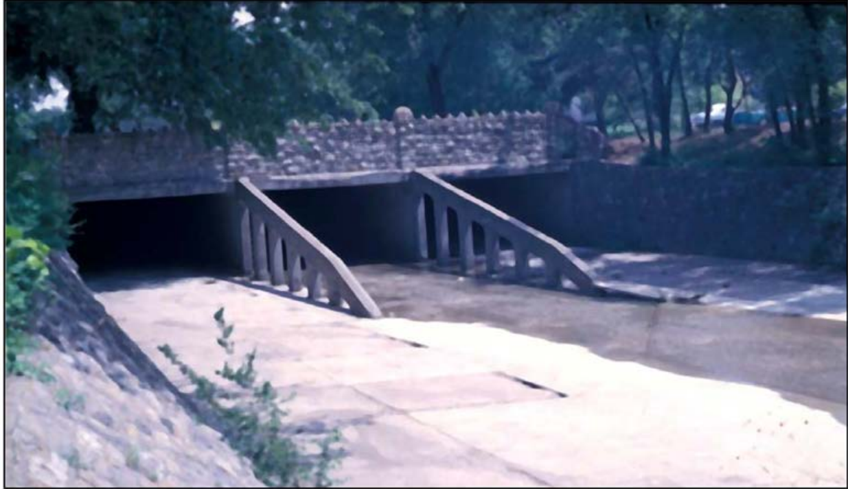
Figure 4-7. Debris Fins Incorporated at Headworks Structure (Example)
