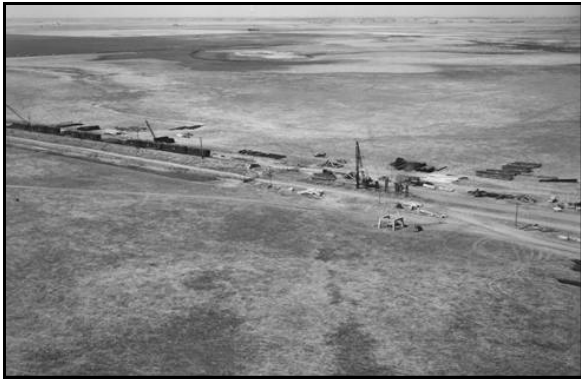
Trestles being rebuilt in 1950s
