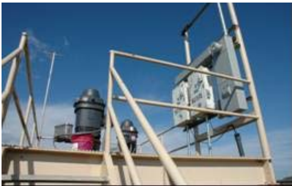
Platform of elevated pump station
