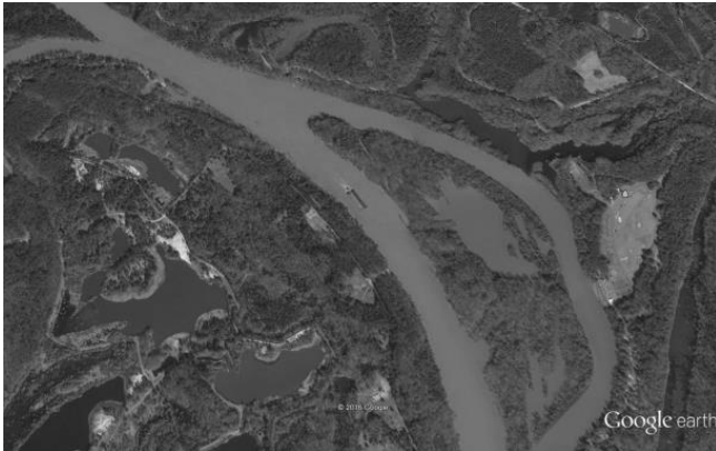
Figure 9.9. Borrow pits (left side of the photo) along the Tennessee–Tombigbee Waterway in Columbus Lake reservoir, Mississippi. Connectivity between these waterbodies and the reservoir varies depending on distance from the reservoir, elevation, and levees but can often be engineered. Photo credit: Google Earth.
