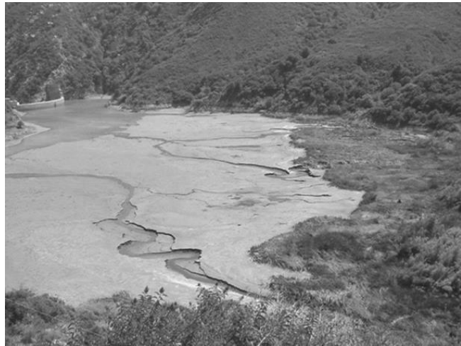
Figure 3.1. Matilija Dam, on the Ventura River Basin, California, was constructed in 1947 and is nearly completely filled with sediment. When constructed, the dam was 190 ft high and impounded a volume of 7,000 ac-ft; by 2015 it was reduced to 400 ac-ft. Photo credit: P. Jenkin.
