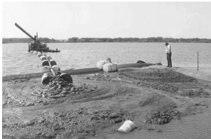
Figure 3.14. The Dry DREdge™ lifts sediment from the reservoir bottom and uses a displacement pump to move it without adding water. The pump fills geotubes with the sediment and then pumps sediment with the consistency of toothpaste behind the tubes to form a small island. Photo credit: J. C. Marlin, Illinois Department of Natural Resources.
