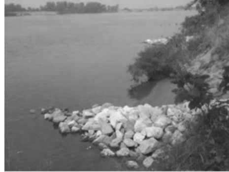
Figure 5.15. Rock vanes at Lost Island Chute, Pool 5, Upper Mississippi River. Photo credit: USACE, Rock Island District.
