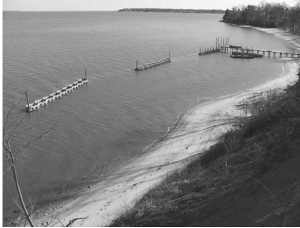
Figure 5.11. Hex-box breakwaters in Potomac River. Photo credit: A. Russo.
