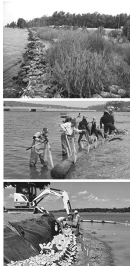
Figure 8.5. General approaches to bank stabilization include live planting, bioengineering, and hard armoring. Photo credits: U.S. Army Corps of Engineers, Savannah District (upper and lower photos), and The Nature Conservancy, Rhode Island (middle).
