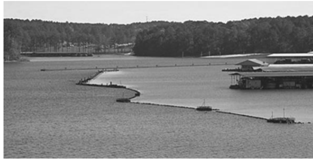
Figure 5.10. View of a floating breakwater, Lake Allatoona reservoir, Georgia. Photo credit: J. Chulick.
