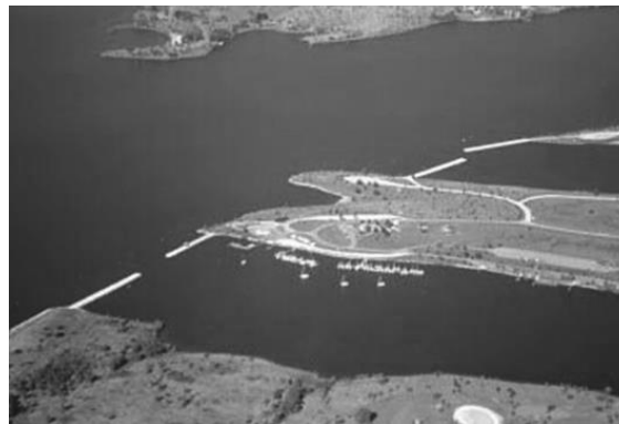
Figure 5.14. Jetties protecting large embayments in Branched Oak Reservoir, Nebraska. Photo credit: Nebraska Game and Parks Commission, Lincoln.
