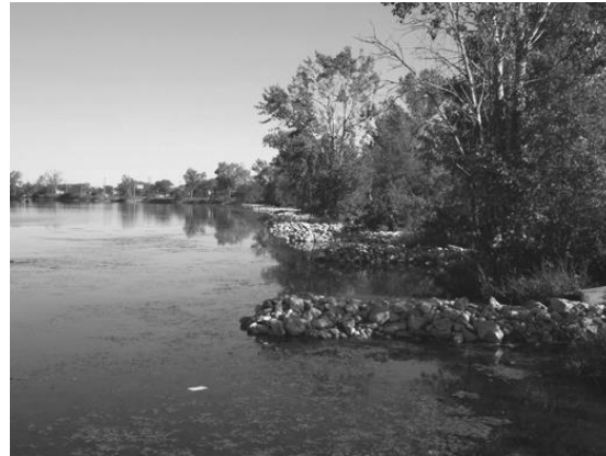
Figure 5.13. Groynes (sometimes referred to as jetties or hardpoints) along a shore of a Nebraska reservoir. Groynes are positioned to reduce nonperpendicular wave energy and allow growth of macrophytes. Photo credit: Nebraska Game and Parks Commission, Lincoln.
