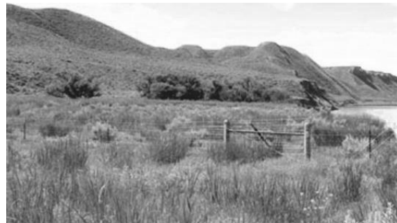
Figure 8.4. Fencing installed to manage grazing along a reservoir in the Missouri River, Montana. Photo credit: Missouri River Conservation Districts Council, Helena, Montana.
