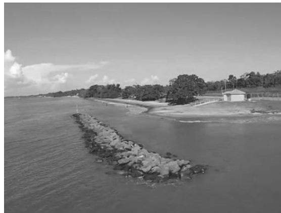
Figure 5.8. Offshore detached breakwater. Photo credit: J. Sullivan, Getty Images.
