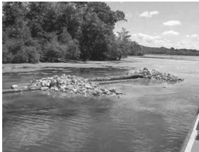
Figure 5.9. Rock-log breakwater at Peterson Lake, Pool 4, Upper Mississippi River. Photo credit: USACE, Rock Island District.
