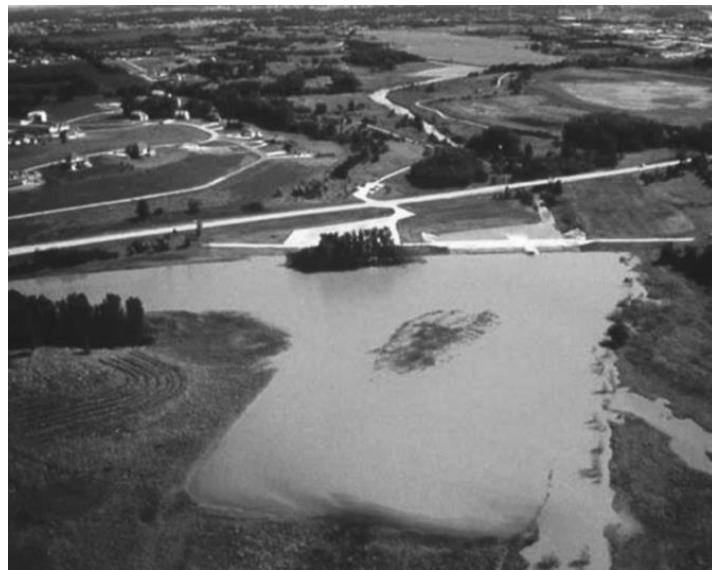
Figure 3.7. Sediment basin constructed above Wehrspann Reservoir, Nebraska, to trap sediment and improve water clarity. Note clear-water reservoir in background. Photo credit: Nebraska Game and Parks Commission, Lincoln.
