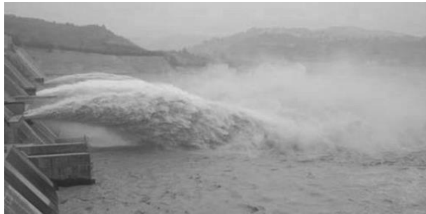
Figure 3.9. Sediment sluicing through a dam in the Yellow River, China. Photo credit: china.org.cn.
