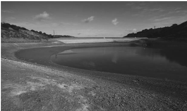
Figure 7.5. Zonation of sediment types caused by fluctuating water levels at Stevens Creek Reservoir, California. Photo credit: J. Sullivan, Getty Images.
