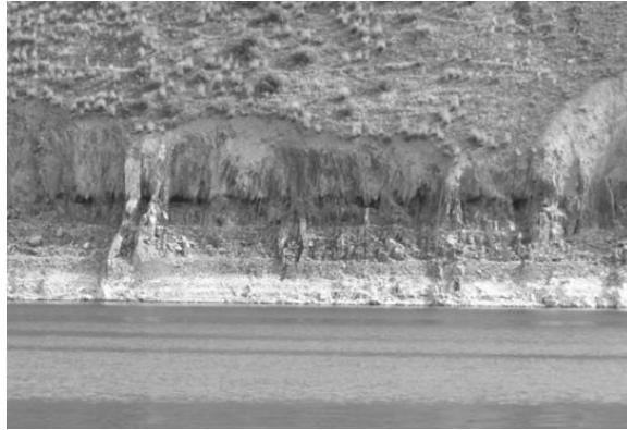
Figure 5.6. Shore erosion is a major source of fish habitat degradation in reservoirs. Erosion not only destroys bank habitat but also blankets substrates with sediment and increases turbidity of the water. In the photo erosion in Brownlee Reservoir, Idaho-Oregon, was caused by seasonal water level fluctuations. Seasonal reservoir operations scour a thin layer of soil from the reservoir "walls." Photo credit: C. Welcker, Idaho Power Company.
