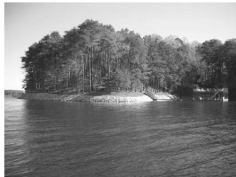
Figure 5.16. Shore revetted with riprap in Lake Lanier reservoir, Georgia, to prevent bank erosion induced by wave action. Photo credit: Marine Specialties, Inc., Gainesville, Georgia.
