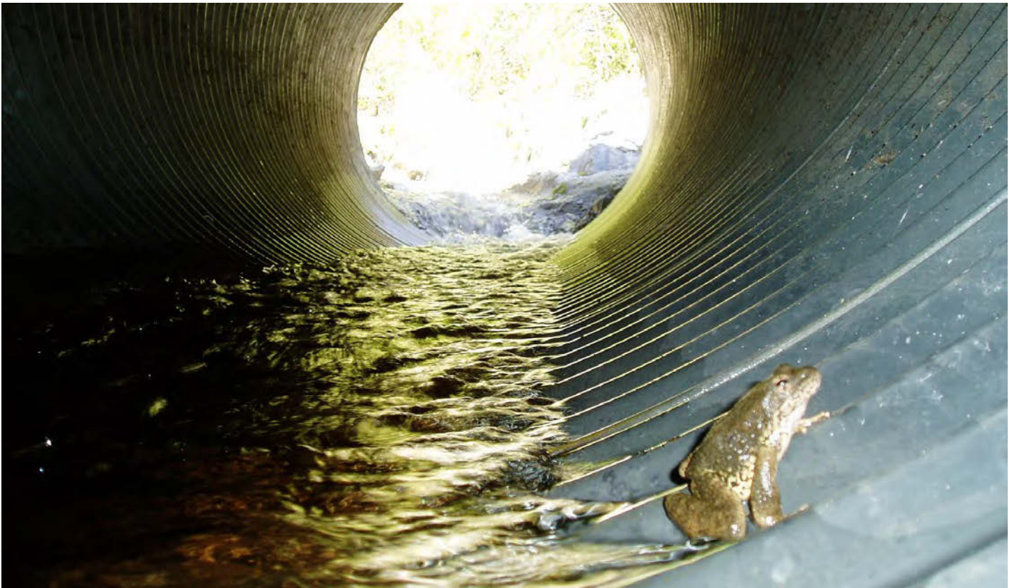
Figure 76: Corrugated culverts without a flat base may be difficult to navigate for some species. Here a foothill yellow-legged frog ( Rana boylei ) can be seen at the side of a corrugated metal passage under Highway 70 at the Shady Rest Area, Butte County, California. Image: Garcia and Associates. See: Garcia and Associates. 2008.
