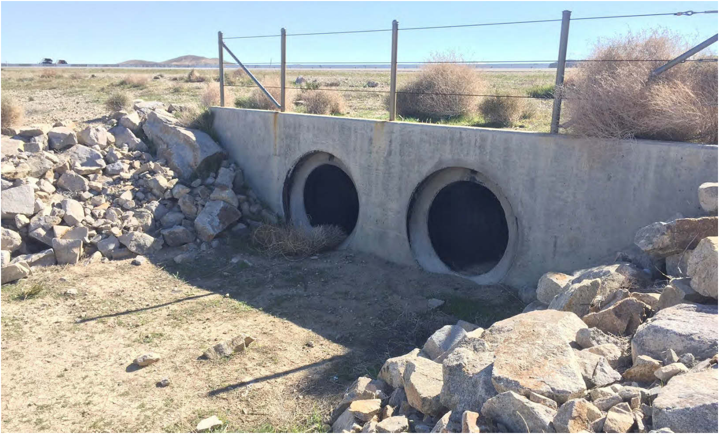
Figure 32: Here two Type 4, 3 ft/90 cm concrete culverts are positioned to accommodate flood events at a desert drainage. Provisions like this might potentially be used by reptiles but many have not been built with directional fencing. They are potentially suitable for modification. Image: Cheryl Brehme
