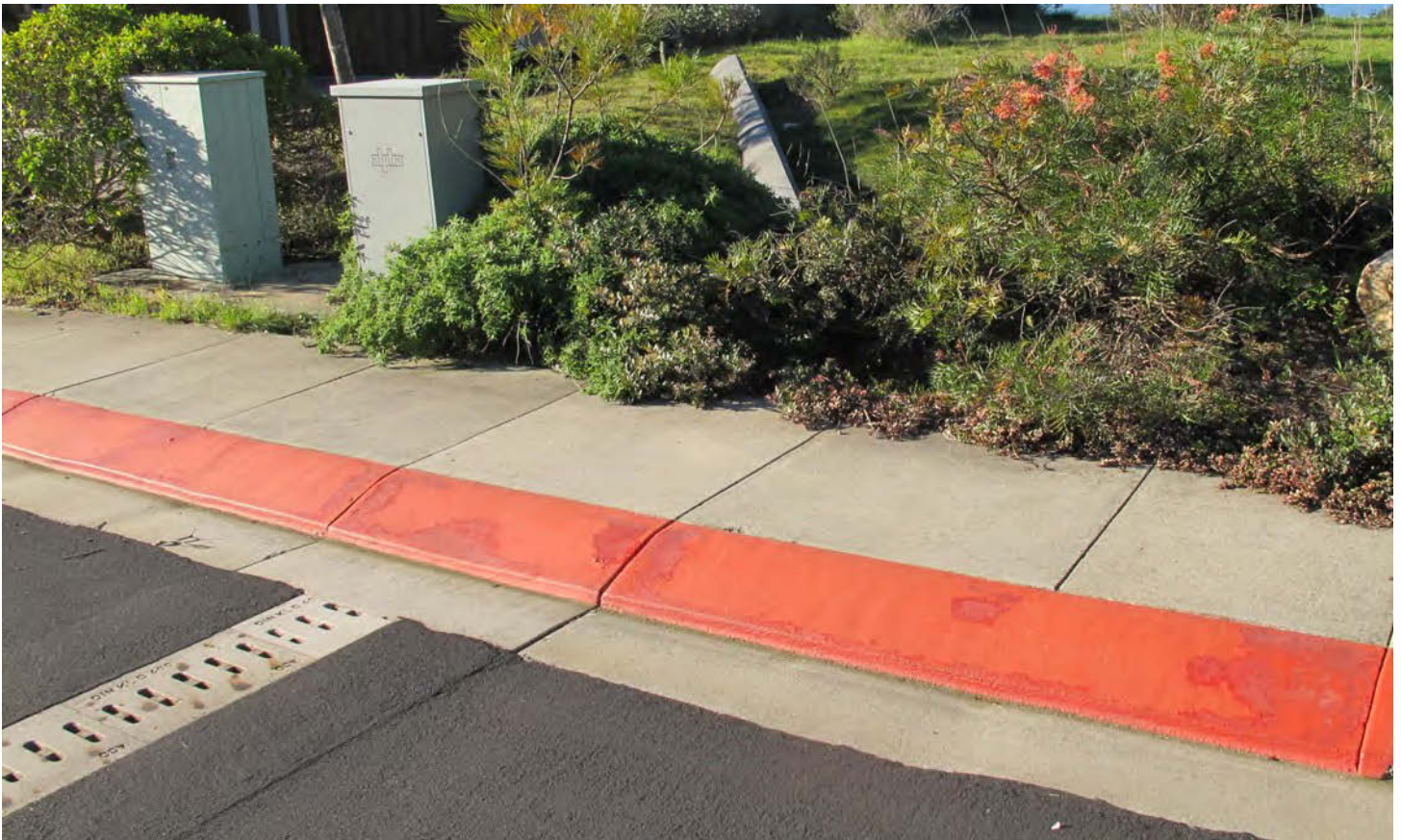
Figure 40: One of several purpose-built slotted polymer concrete surface passages (bottom left) built in 1999 for the Santa Cruz long-toed salamander at Seascapes Uplands, Santa Cruz. These were constructed along with short sections (center, running up slope) of one-way plastic panel fencing to try to minimize construction impacts on houses and the gardens that remain a part of the salamander's terrestrial habitat. Image: Tom Langton
