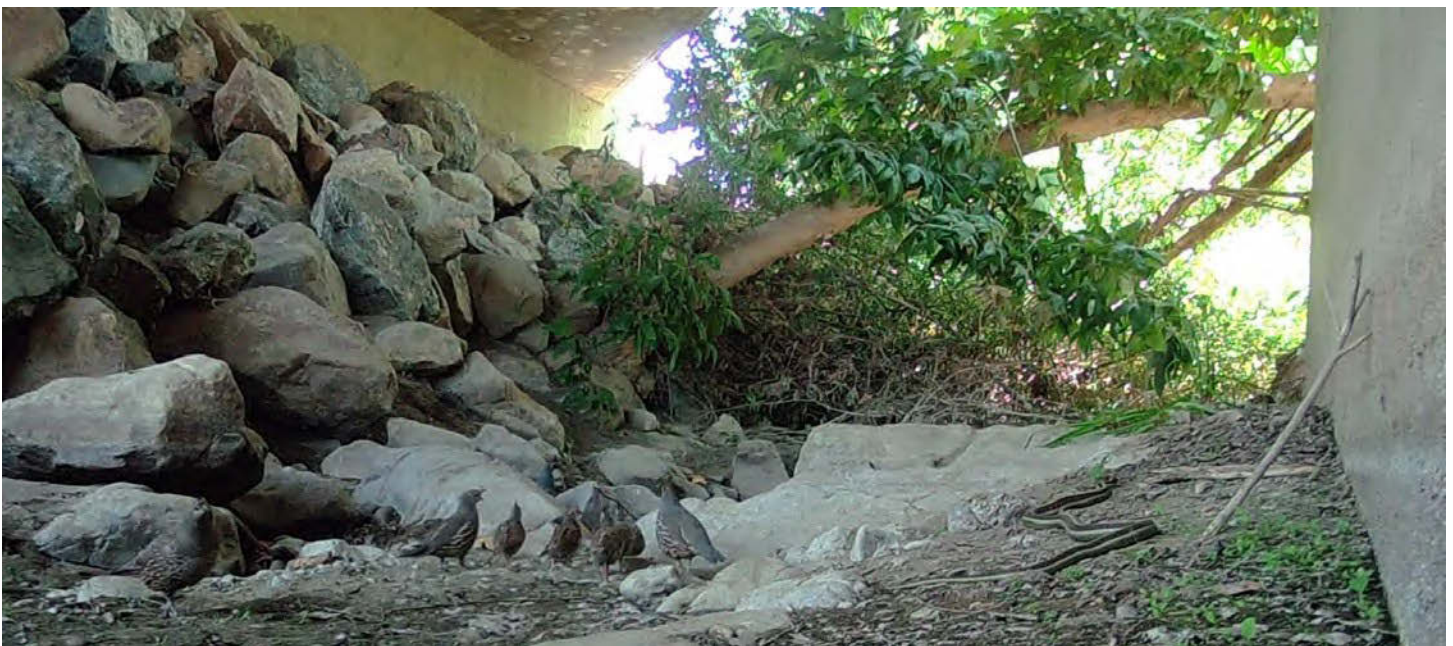
Figure 25: An adult garter snake is using a Type 3 structure on State Route 152 in California. This bridge spans Pacheco Creek near San Felipe Lake on the Pacheco Pass Highway near Gilroy. California quail ( Callipepla californica ) are also present. Image: Pathways for Wildlife, Santa Clara County, CA.
