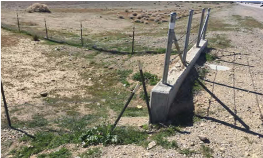
Figure 53: Fine wire mesh tortoise fencing (barely visible in photograph) on metal posts along Interstate 15 in San Bernardino County, located within desert habitat at a culvert underpass. Image: Cheryl Brehme
