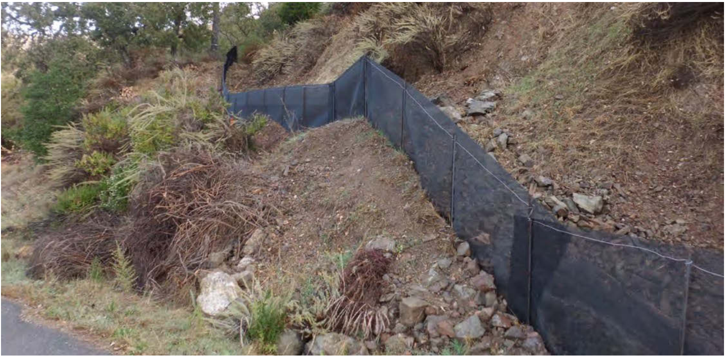
Figure 50: A rigid monolithic plastic (HDPE) mesh fence with overhang. Fine holes of under 0.2 in/5 mm) give a degree of visibility through them. These are often seen on construction sites but should not be confused with fences designed for permanent road and rail crossing systems. Image: Vince Morris
