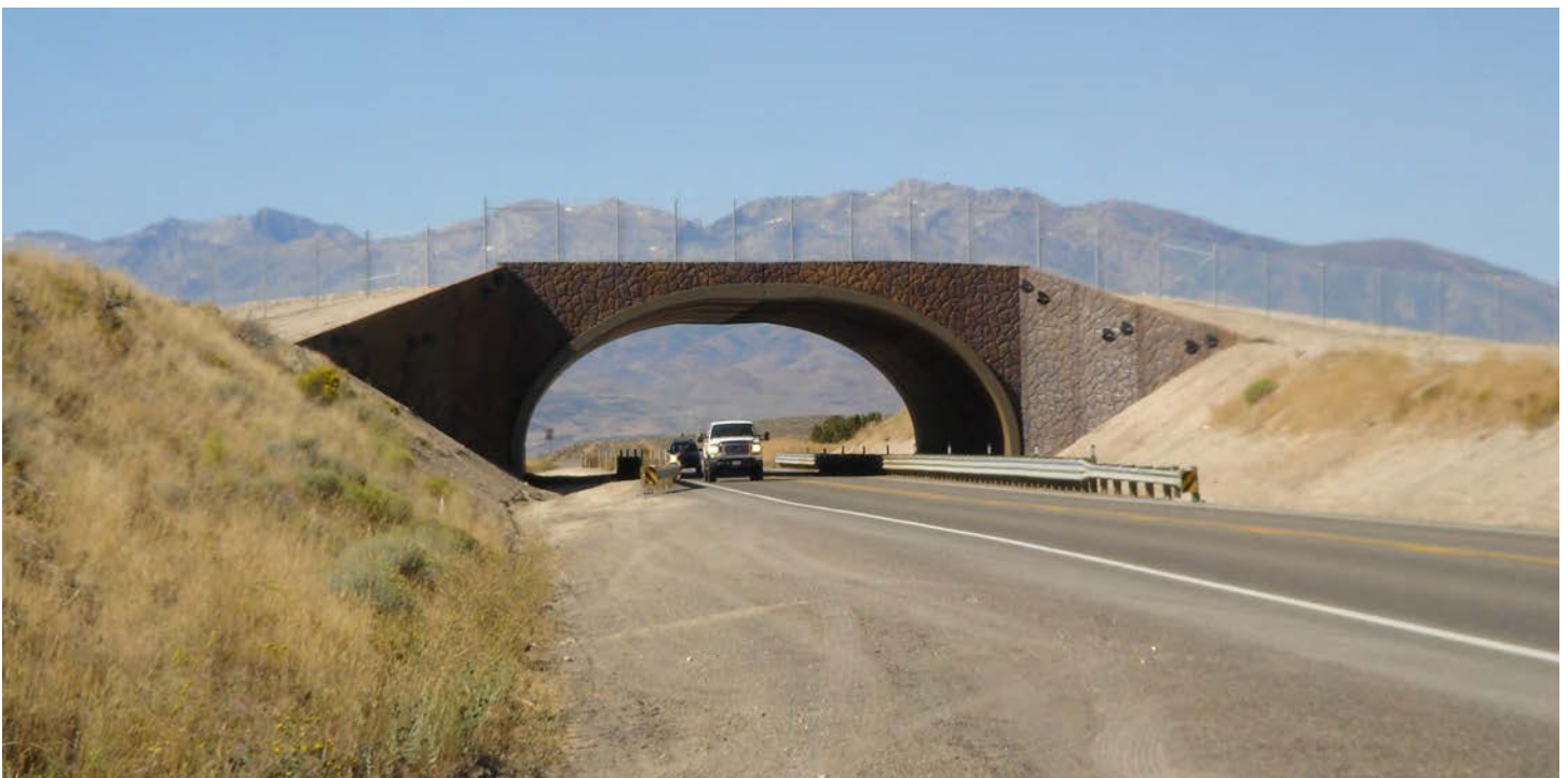
Figure 19: Type 1C wildlife overpass that is 150 ft/46 m wide and was constructed specifically for mule deer on Highway 93 north of Elko, Nevada. Image: Nevada Department of Transportation
