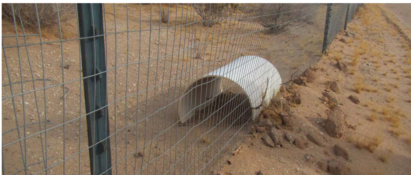
Figure 64: This shade structure is made from a 12-14 in PVC pipe tied to the fence. Tortoises may die from heat-stress when pacing a mesh fence line where no shade is available. Image: Cheryl Brehme.
