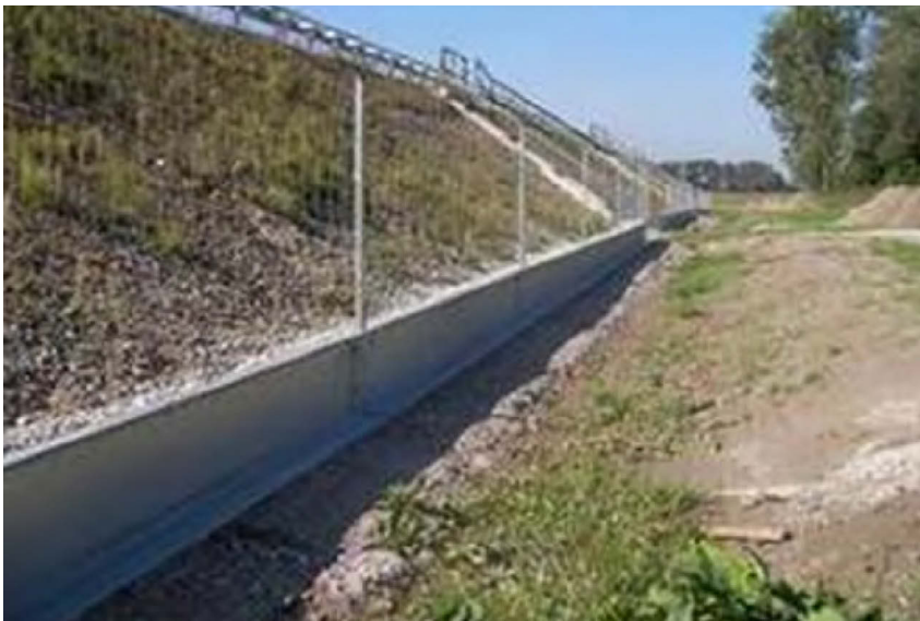
Figure 57: Dual purpose permanent barrier for deer and small animals. The tall deer mesh fence with metal support poles is built together with a small galvanized steel animal guide wall with an overhang. Image: ACO
