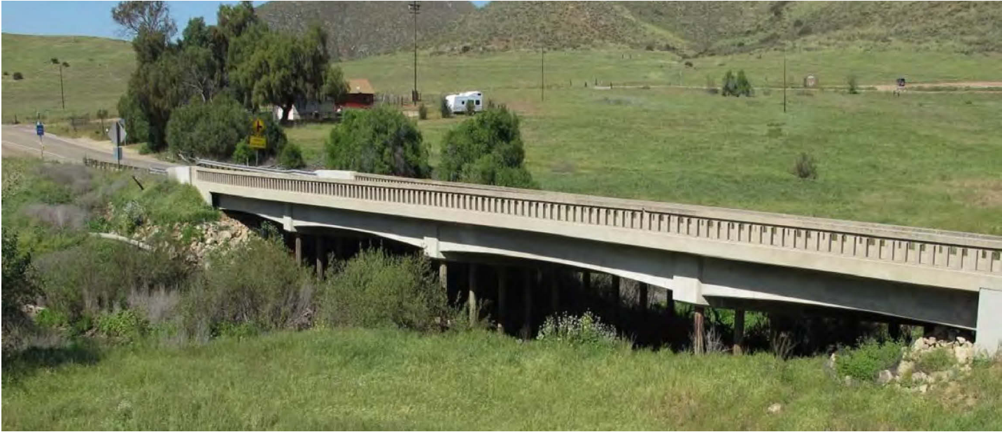
Figure 23: Image shows a Type 2 bridge that is about 120 ft/36.5 m in length. This bridge is located over a stream at the junction of Campo Road with Honey Springs Road and Otay Lakes Road, San Diego County. Image: Tom Langton
