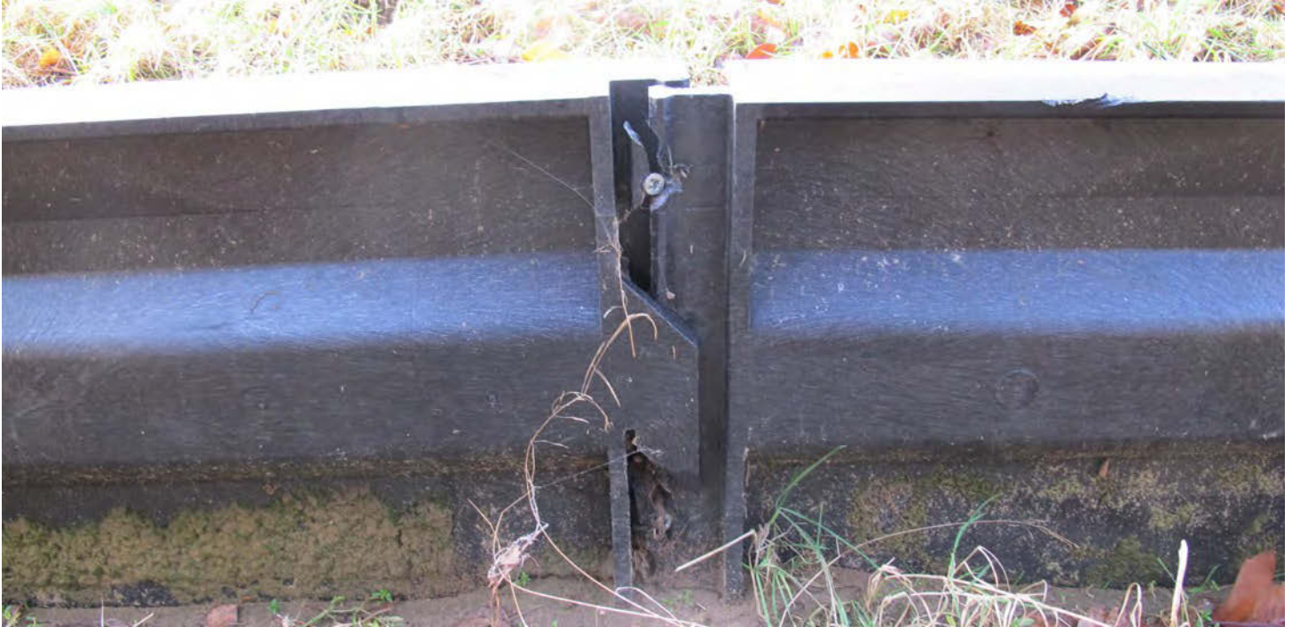
Figure 52: Some types of cast plastic barrier may expand and contract in heat and sunlight, causing problems for joints. Fixings should be constructed to allow space for such movements.
