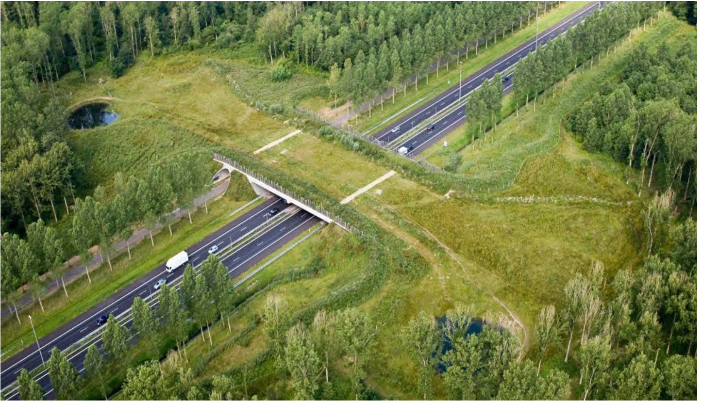
Figure 20: Type 1C wildlife overpass with emphasis on amphibian connectivity (Netherlands). Features include a narrow wet strip along the length of the passage connecting small ponds at each end. Image: Rijkswaterstaat.
