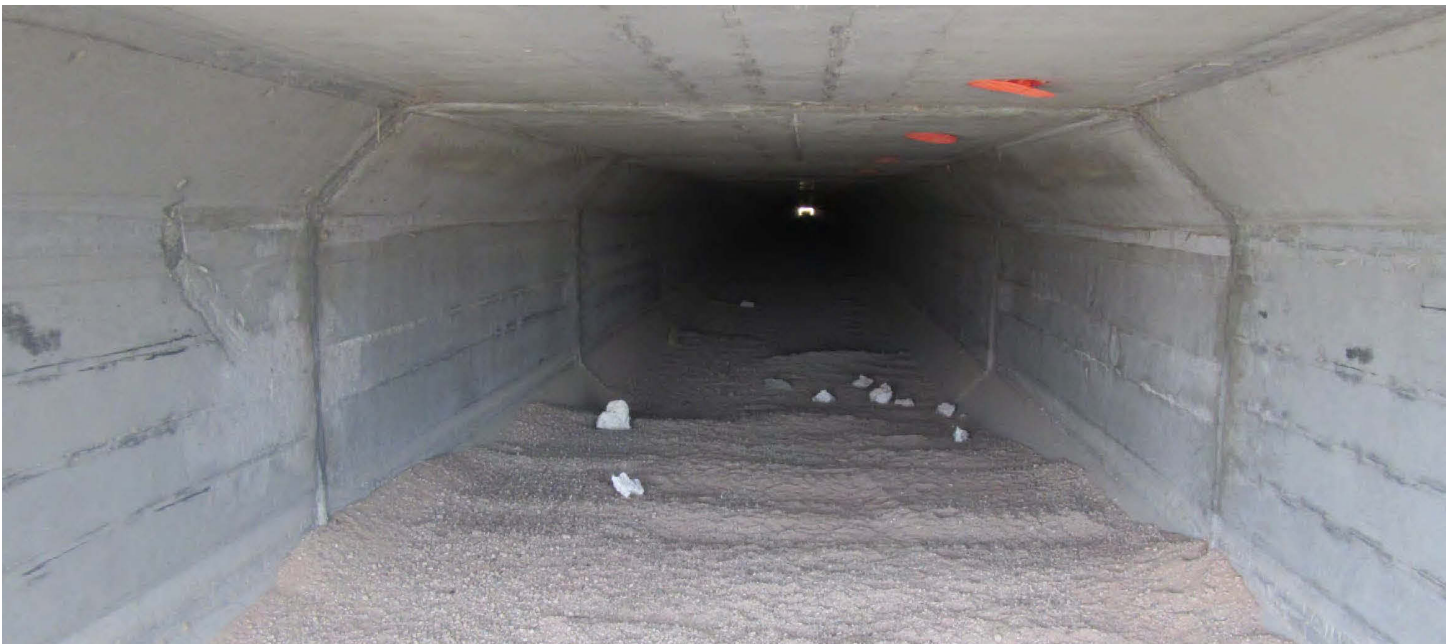
Figure 29: With a large median and easements under a four-lane highway, desert culverts can be extremely long (over 300 ft /90 m) and dark during the day. The view foreground here is lit by a camera flash.
