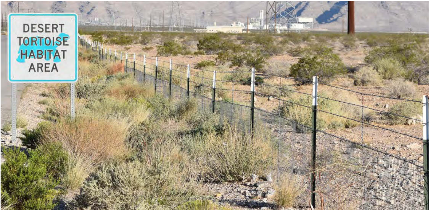
Figure 54: Typical wire mesh and stock fencing on metal posts in desert tortoise habitat. Image: Dean Swenson
