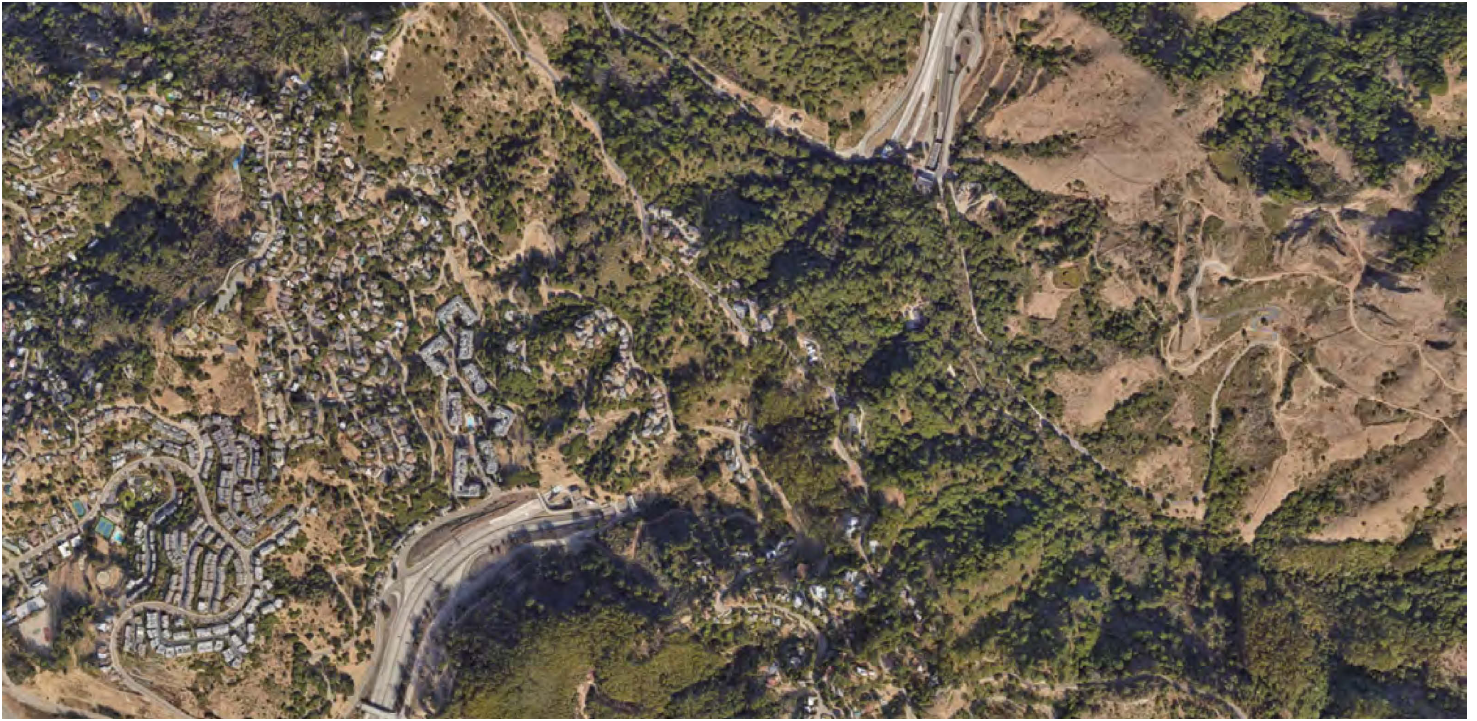
Figure 16: The Caldecott Tunnel is located on Highway 24, near Oakland, Caltrans in District 4. Tunneling for about 3,300 ft/1000 m, helped to protect the area known as the Caldecott Wildlife Corridor (East Bay Regional Park District), preserving a movement corridor for wildlife between Oakland and Orinda. Image: Google Maps.
