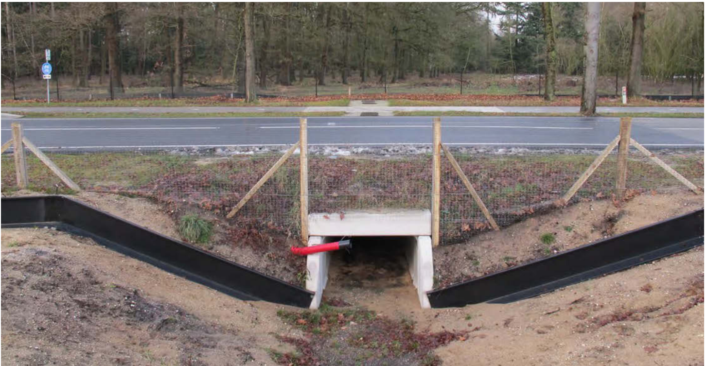
Figure 30: This is a Type 4 cast concrete 'bottomless' or 'stilt' passage with side walls built on foundations in the Netherlands. It is constructed below a two-lane road with cycle path, particularly to enable rare lizard dispersal. The sandy base substrate is in contact with the natural water-table. Image: Tom Langton
