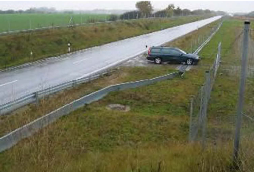
Figure 58: Here, a free-standing metal fence and a large mammal fence separate in order to go around a road over-bridge that runs perpendicular to the main highway. Note a 'stop grid' beneath the car. The deer fence also has a gate positioned in front of the point at which the car (and agricultural vehicles) can enter the surrounding landscape. Image: Tom Langton
