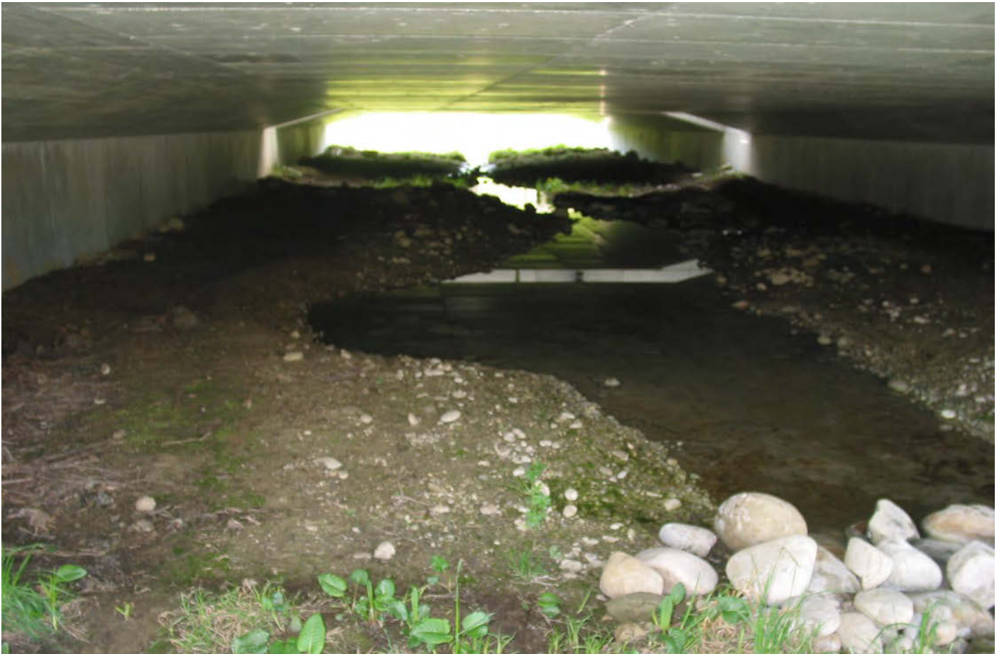
Figure 37: A Type 4 purpose built passage with a light and air gap in the median and with wet and damp conditions suitable for amphibians and other wildlife that prefer damp conditions. Image: Andreas Meyer, KARCH
