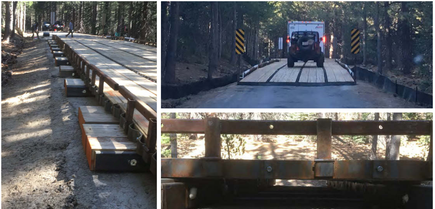
Figure 43: Experimental raised micro-bridge for the Yosemite toad ( Anaxyrus canorus ) in the Sierra National Forest. Images show 'safe space' and directional fencing to help guide animals to the underpass. Images: Cheryl Brehme
