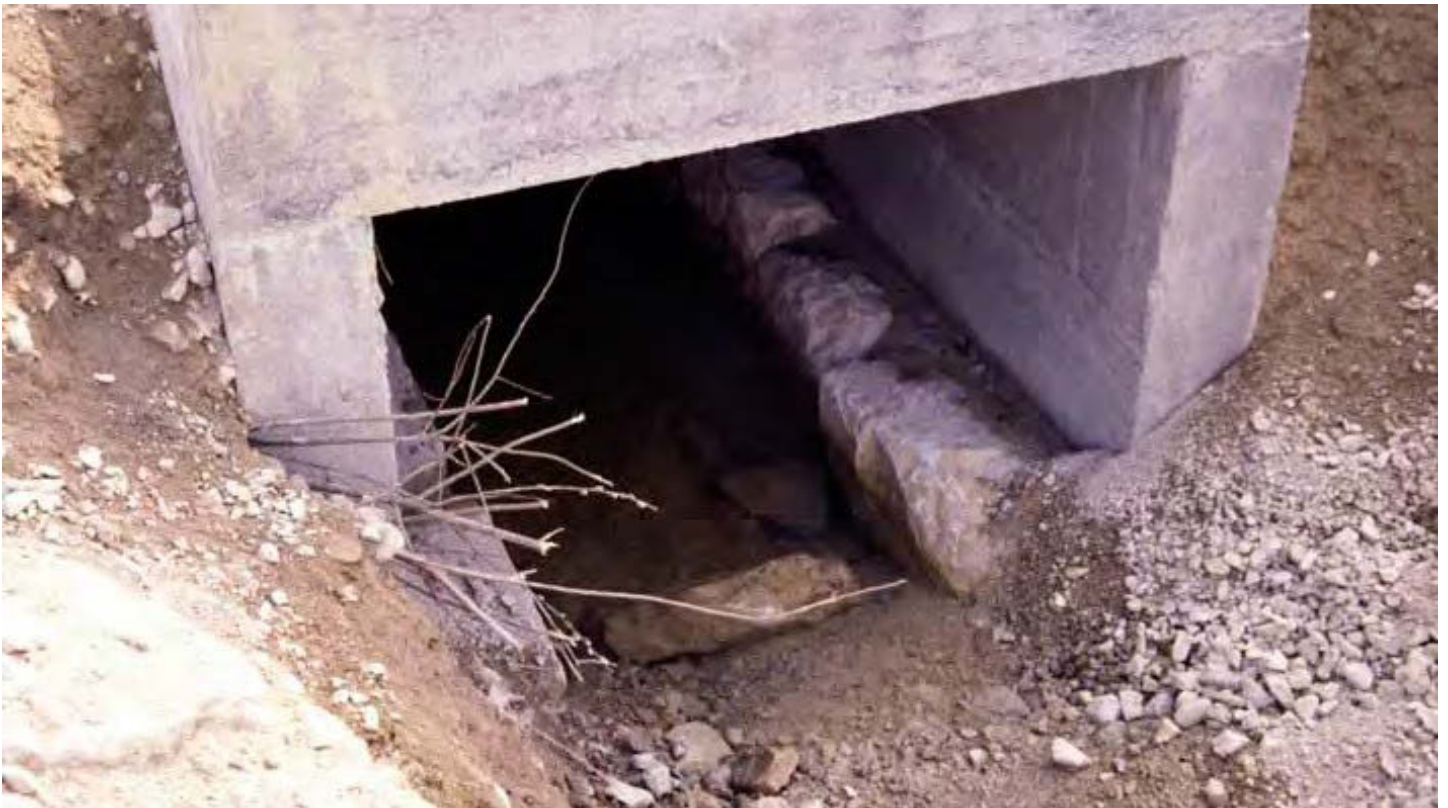
Figure 36: A Type 4 sized passage with dry ledges, in addition to a central wet channel is suitable for a range of species, shown here at a wildlife crossing in central Europe. Image: Silvia Zumbach, KARCH
