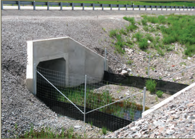
Photo 22. 3.4 m x 2.4 m tunnel on Highway 69. © K. Gunson
