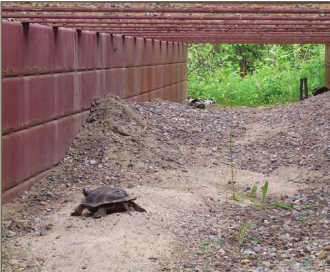
Photo 54. Wood Turtle using open-grate tunnel © A. Mui
