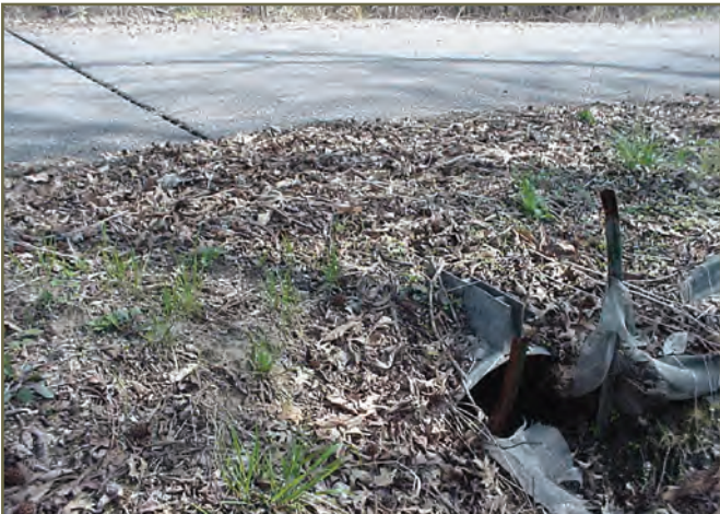
Photo 16. Pipe culvert with slotted top installed for Timber Rattlesnakes in Illinois, U.S. © S. Ballard
