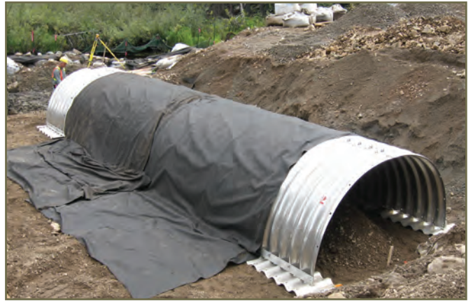
Photo 15. Aluminum arch culvert on metal footings. © K. Williams
