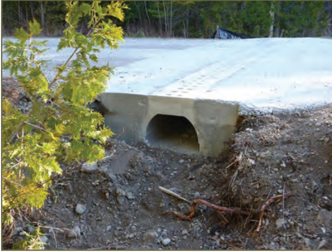
Photo 30. Earth excavated to allow at grade entrance to tunnel. © D. Filip
