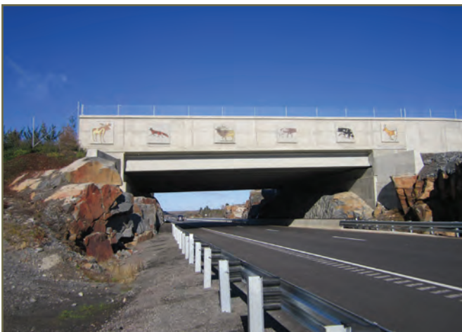
Photo 26. Wildlife overpass on highway 69 showing rock footing K. Gunson.
