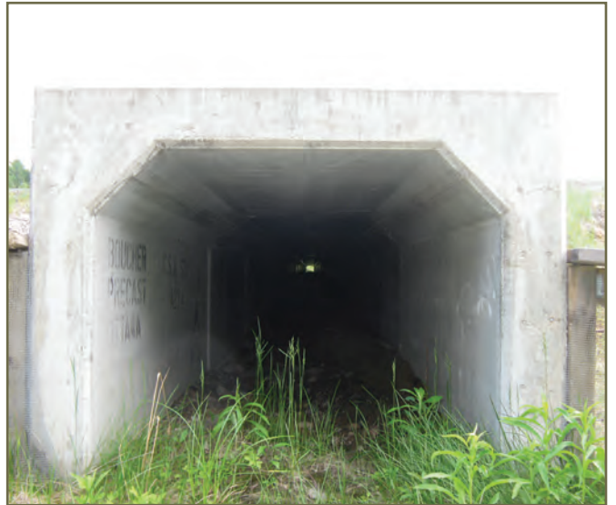
Photo 4. Open-bottom tunnel along highway 69, Ontario. © K. Gunson
