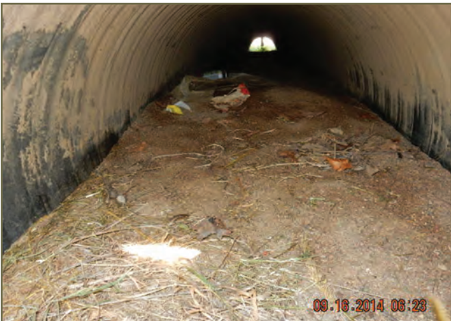
Photo 18. Buried plastic round culvert allowing terrestrial flat floor in Sweden © K. Gunson
