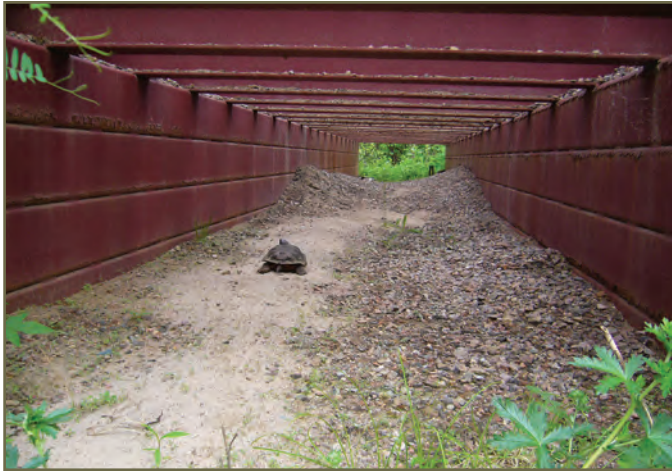
Photo 35. Turtle using open-grate tunnel with natural substrate at bottom © A. Mui
