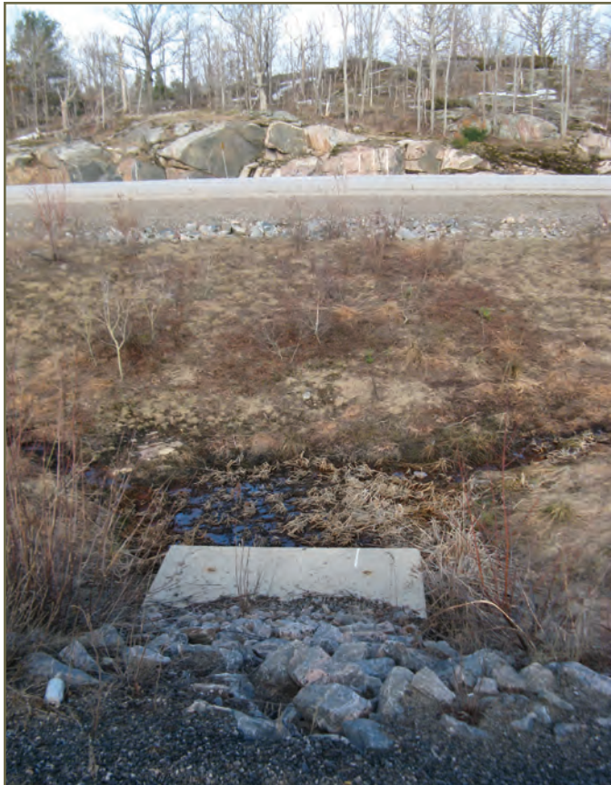
Photo 27. Drainage box tunnel left open in median along highway 69 © K. Gunson
