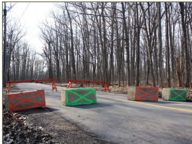
Photo 55. Road Closure on King Road, Halton Region. © N. Finney
