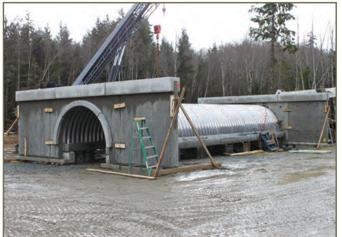
Photo 19. Arch culvert preassembled off site © K. Williams
